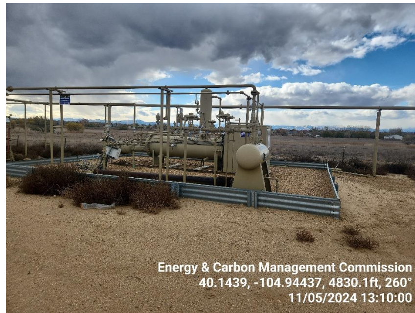
Photo 4 Horizontal heated separator.
