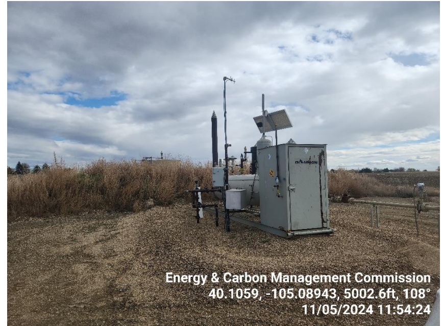
Photo 6 Horizontal Heated Separator.
