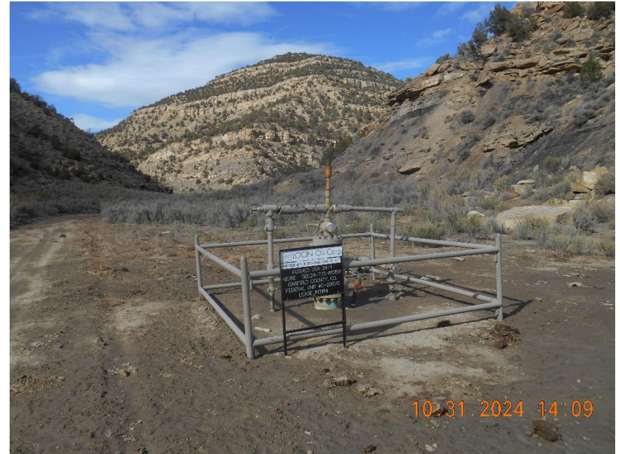
Wellhead with sign and fence
