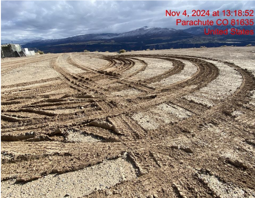
Lack of Stabilization – Photo #04699
