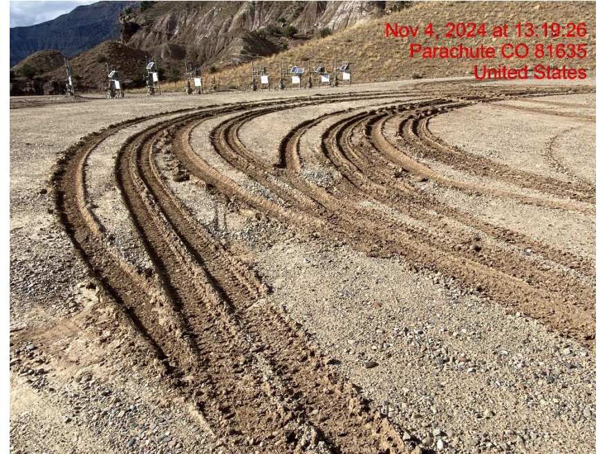
Lack of Stabilization – Photo #04700
