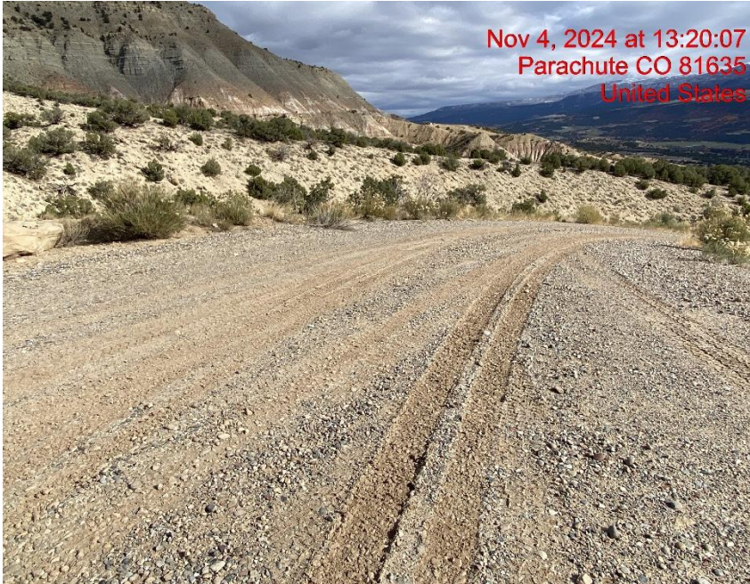
Insufficient Tracking BMPs – Photo #04702
