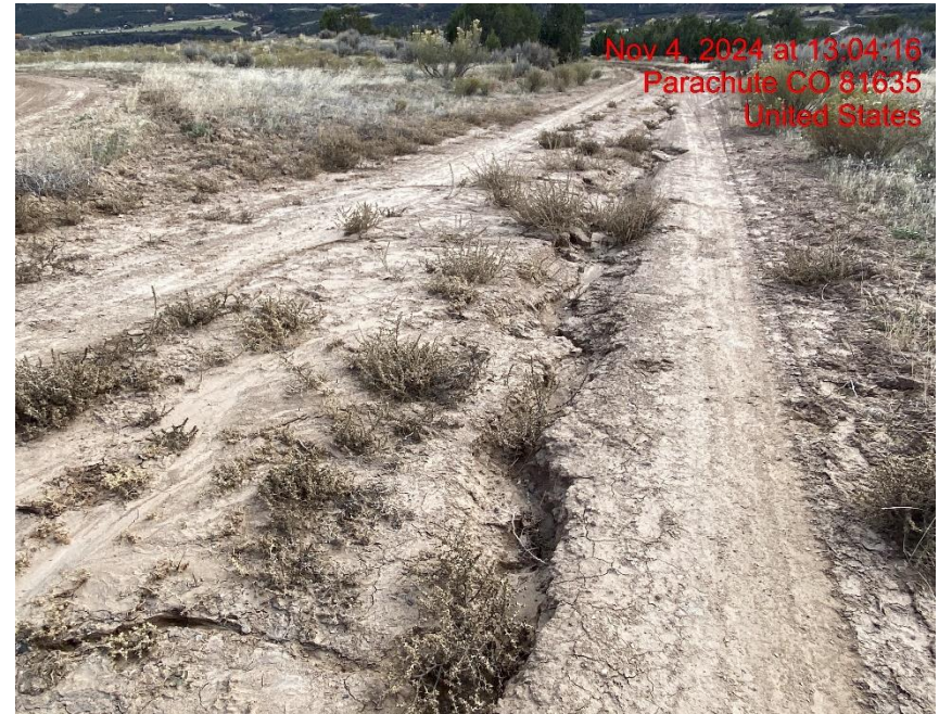
Rill Erosion in Access Road – Photo #04692
