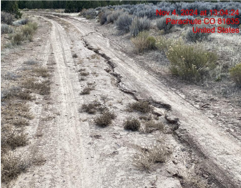
Rill Erosion in Access Road – Photo #04693
