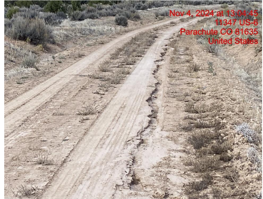
Rill Erosion in Access Road – Photo #04694
