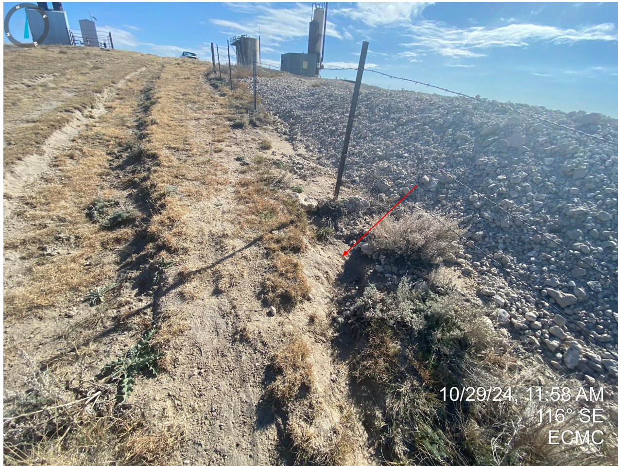
Photo 6. Erosion degradation on north side of pit.
