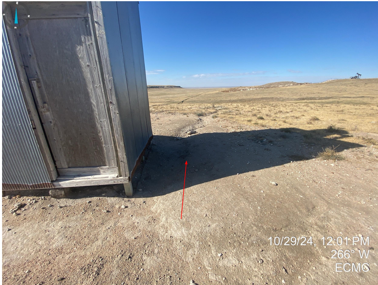
Photo 10. Erosion degradation observed on northside of meter shed.
