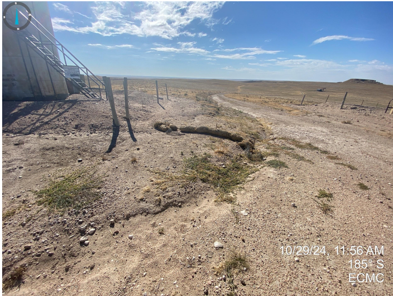
Photo 1. Erosion degradation observed around the production areas. Degraded straw wattle appears to have been reinstalled, however, it does not appear to have been installed per good engineering practices (e.g. trenched and backfilled) and is not properly function in its current state.
