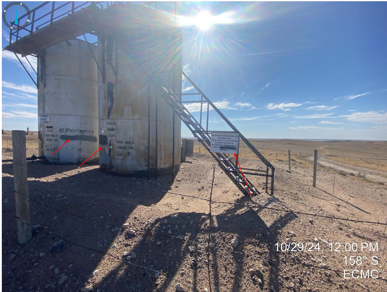
Photo 8. No emergency contact information/number posted at the tank battery.
