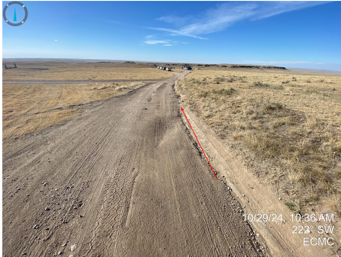
Photo 2. Erosion degradation observed along the access road.
