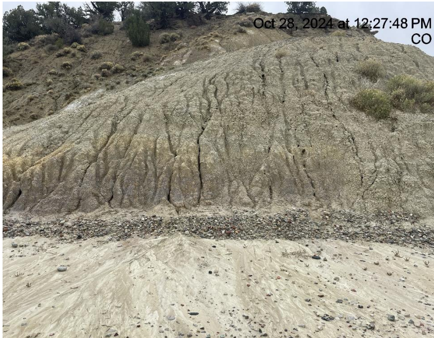
Photo # 7544 Erosion & transport of sediment onto lease road/insufficient BMP's (approximately 2/10 th of a mile from entrance to location)
