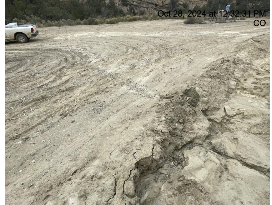
Photo # 7547 Tunnel erosion & transport of sediment onto lease road/BMP's need maintenance (approximately 3/10th of a mile from entrance to location)
