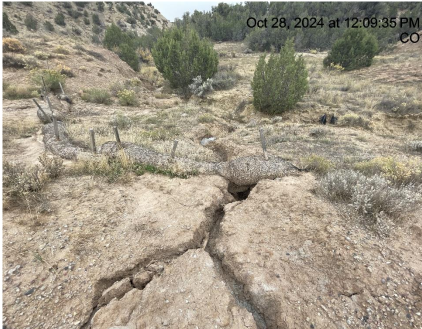
Photo # 7540 Failure to minimize erosion & transport of sediment/BMP's need maintenance
