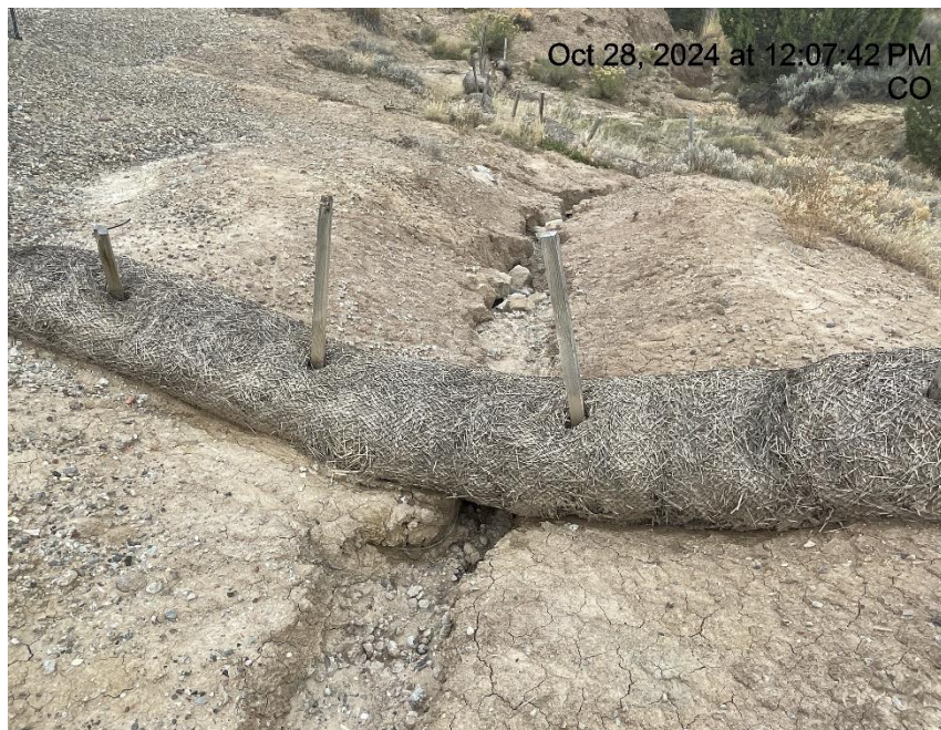
Photo # 7542 Failure to minimize erosion & transport of sediment/BMP's need maintenance
