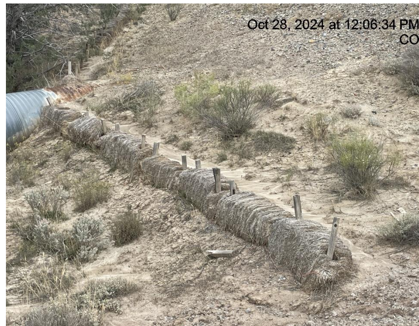
Photo # 7549 Large amount of sediment buildup at hay bales /BMP's may need maintenance in near future (Off edge of lease road near entrance to location)
