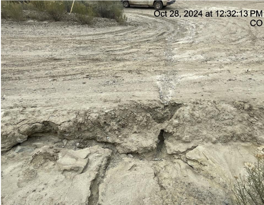
Photo # 7546 Tunnel erosion & transport of sediment onto lease road/BMP's need maintenance (approximately 3/10th of a mile from entrance to location)
