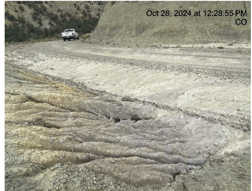
Photo # 7545 Erosion & transport of sediment onto lease road/insufficient BMP's (approximately 2/10 th of a mile from entrance to location)
