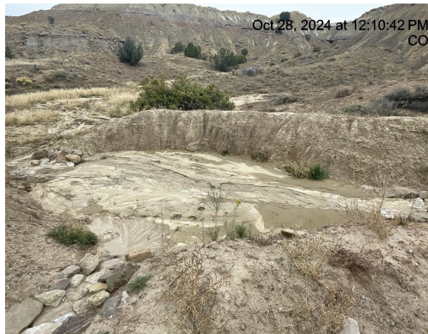
Photo # 7543 Sediment trap needs maintenance (S/SW corner of location near entrance to location)
