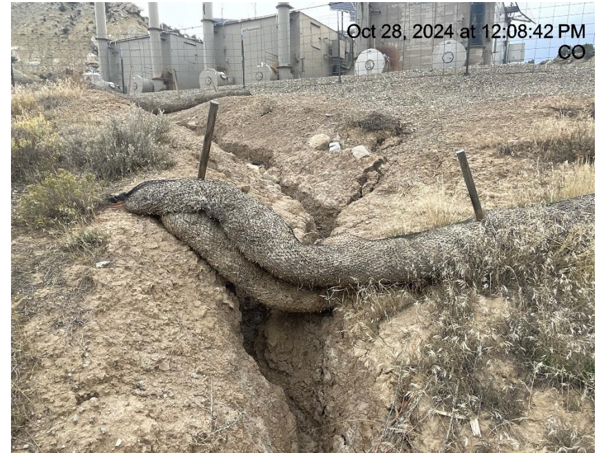
Photo # 7541 Failure to minimize erosion & transport of sediment/BMP's need maintenance
