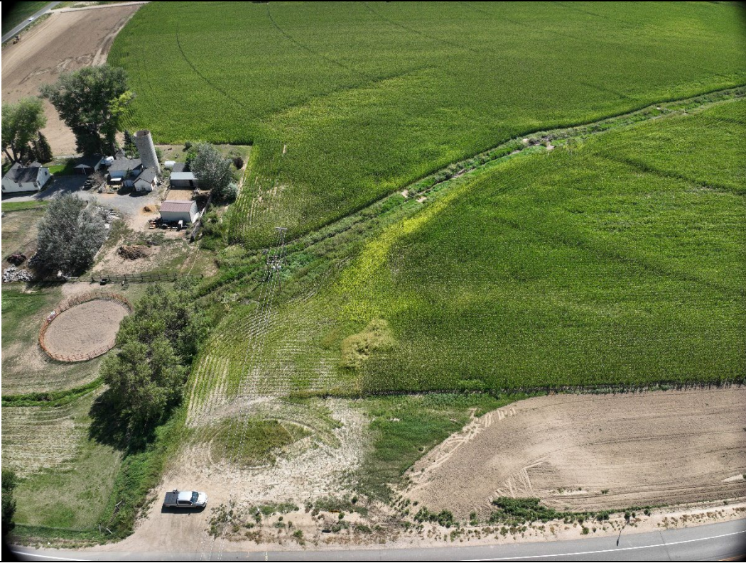
In View – Tank Battery (Loc ID 463217 ), Flowline, Municipal Water Pipeline Construction Impact SOUTH – 40.349315 / -104.945659
