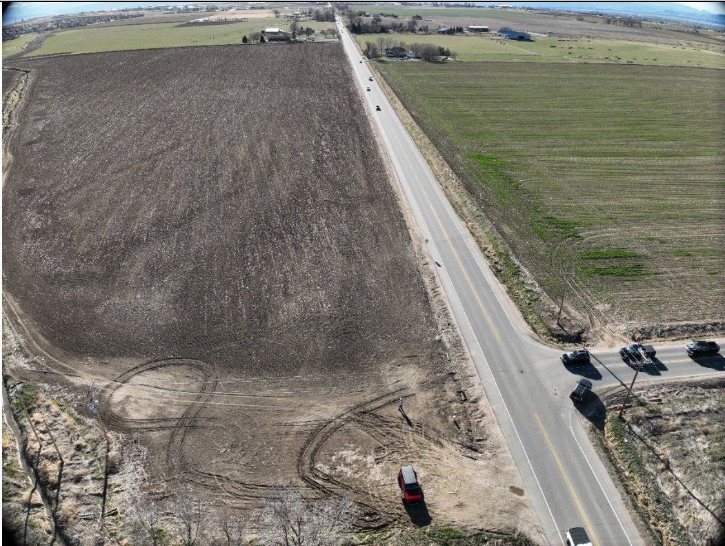
In View – Well, Tank Battery (Loc ID 463217 ), Flowlines
