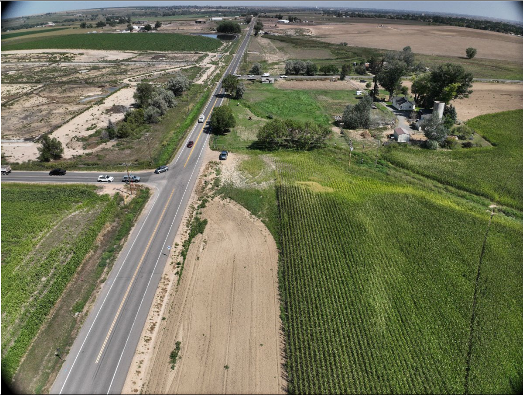
In View – Tank Battery (Loc ID 463217 ), Flowlines, Municipal Water Pipeline Construction Impact EAST – 40.348877 / -104.946819
