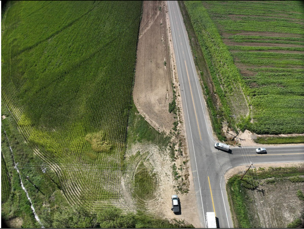
In View – Tank Battery (Loc ID 463217 ), Access Road, Flowline WEST – 40.348937 / -104.945030
