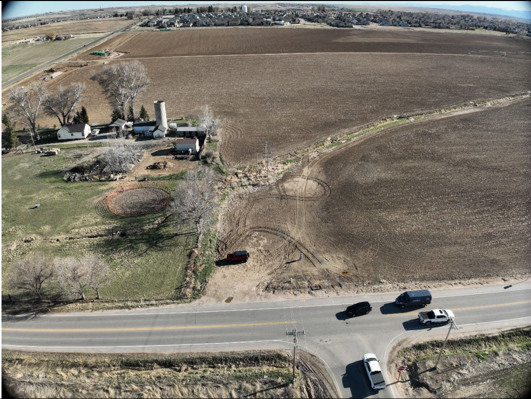
In View – Tank Battery (Loc ID 463217 ), Flowlines
