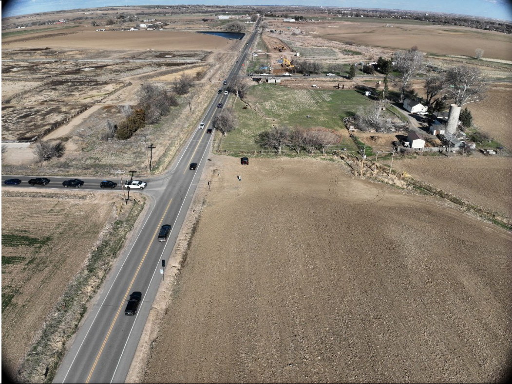
In View – Tank Battery (Loc ID 463217 ), Flowlines
