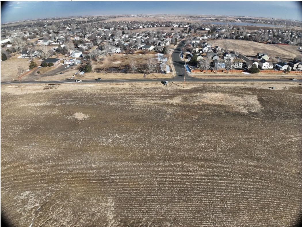
In View – Tank Battery, Access Road, Flowline
