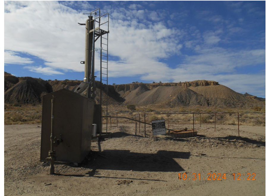
Meter housing and Dehydrator with blowdown tank
