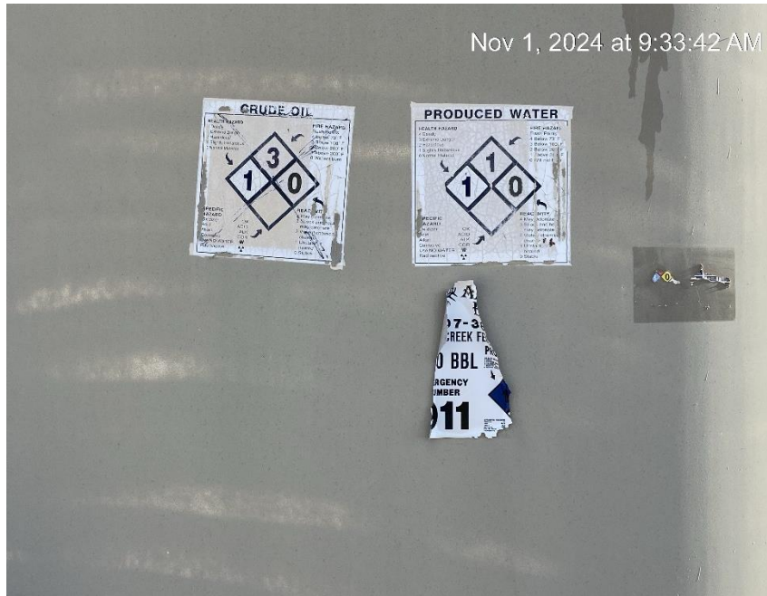
Production tank missing required labels
