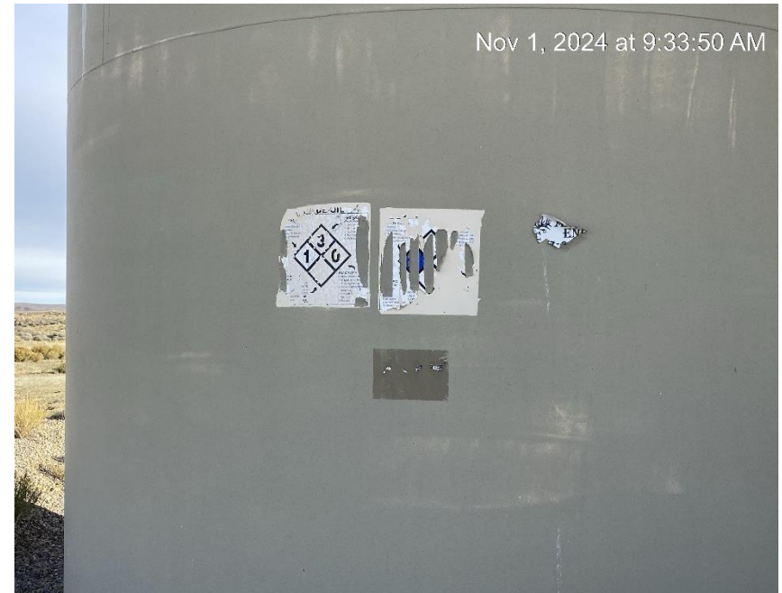
Production tank missing required labels
