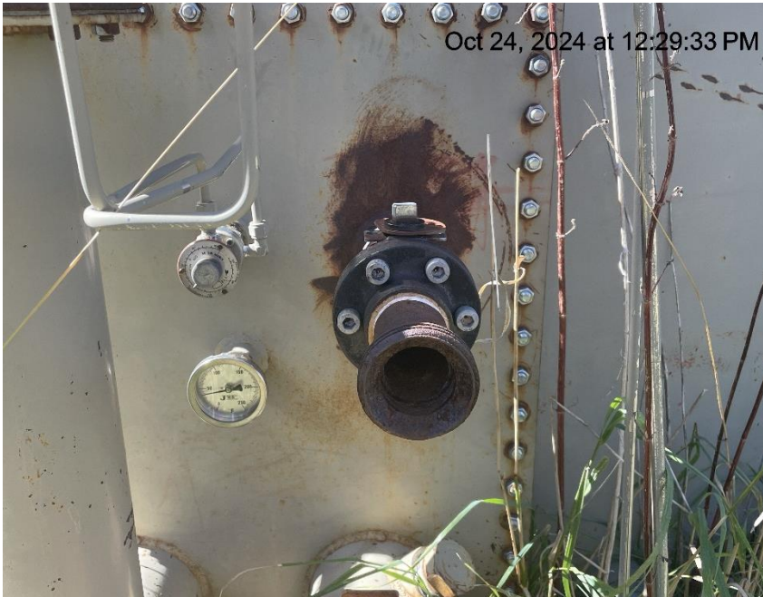
Photo # 7071 Open ended load line
