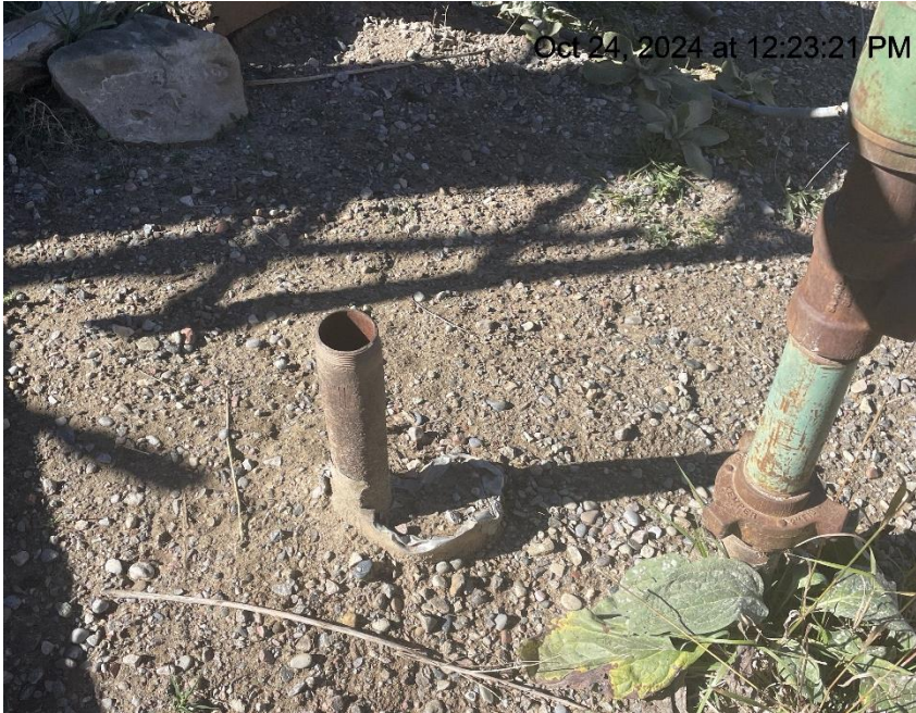
Photo # 7069 Open ended piping/available for entry by wildlife/wildlife hazard
