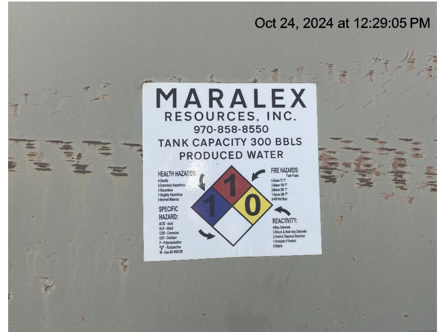
Photo # 7068 Tank label contains inaccurate info/does not comply with CECMC rules
