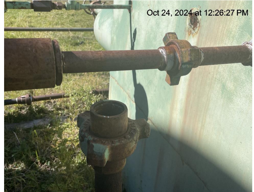
Photo # 7070 Open ended piping/available for entry by wildlife/wildlife hazard
