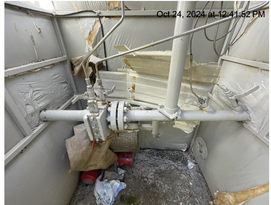
Photo # 7072 Meter calibration info not conspicuously posted
