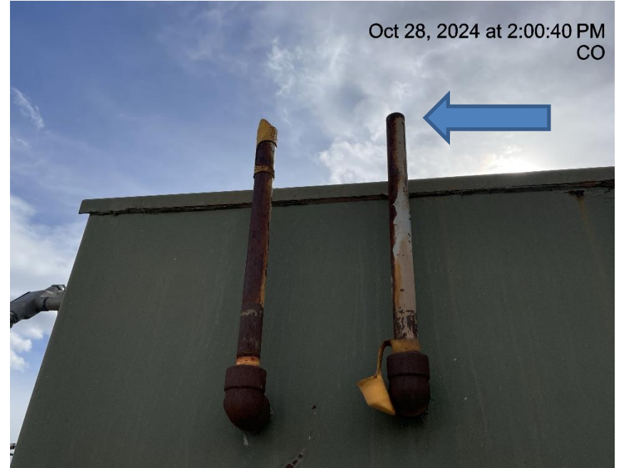
Photo # 7759 Rupture disc vent line does not comply with CECMC pressure safety device rules
