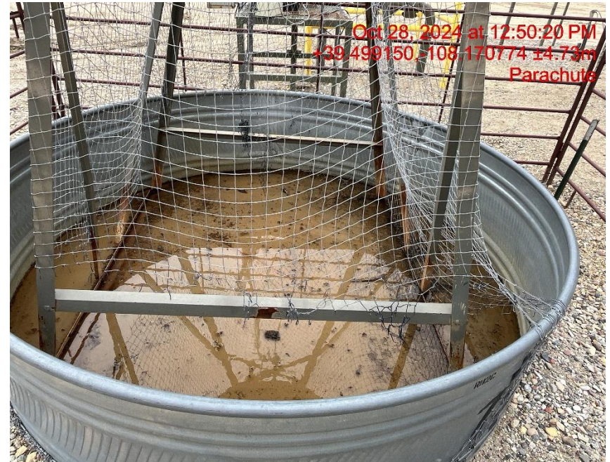
Photo # 8166 Wildlife protection for methanol tank containment needs maintenance/netting is damaged/wildlife hazard
