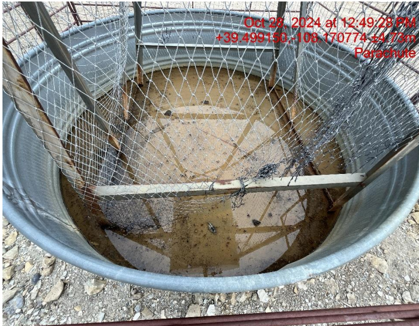
Photo # 8163 Wildlife protection for methanol tank containment needs maintenance/netting is damaged/wildlife hazard
