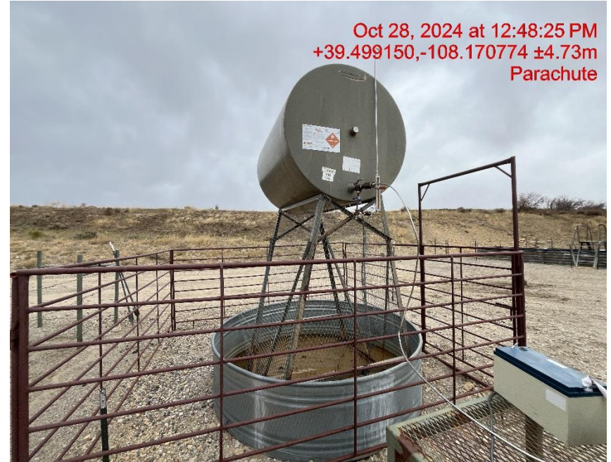
Photo # 8159 Wildlife protection for methanol tank containment needs maintenance/netting is damaged/wildlife hazard
