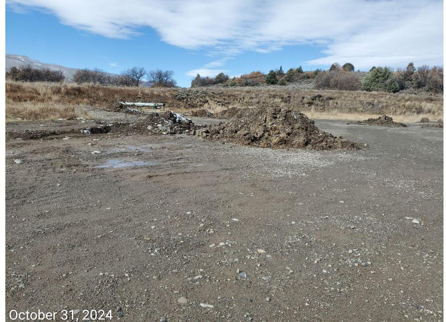
**Photo 2:** Photos 2-3 examples showing excavations missing required fencing, and stockpiled soils missing BMPs pursuant to Rules 1002.c and 1002.f.
