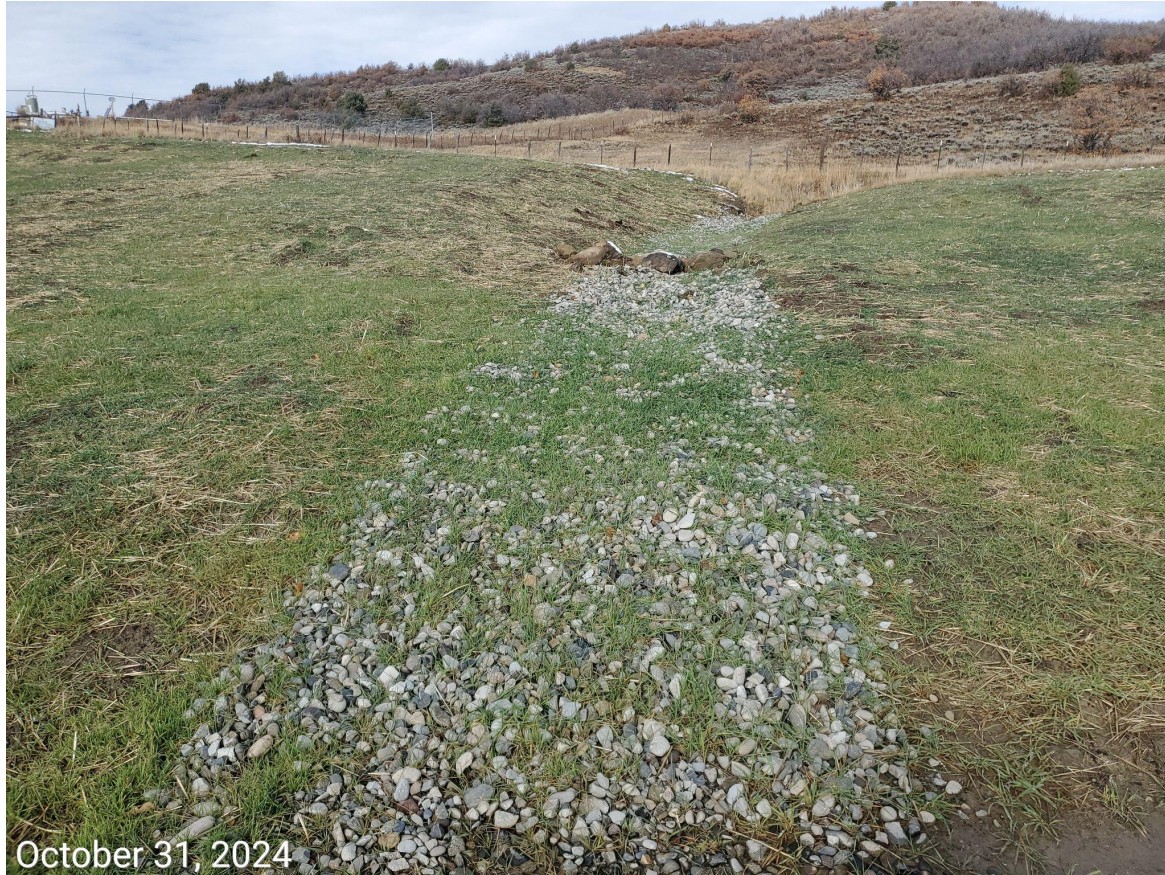
Photo 5: Photo taken from the north end of the Location, facing north. Photo shows erosion degradation at the culvert outlet has been repaired.
