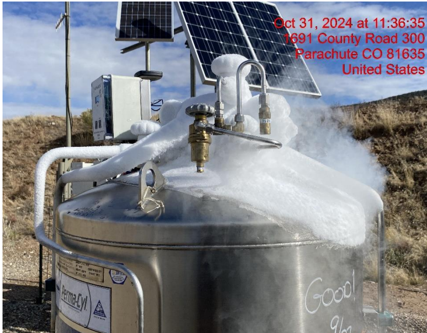
Nitrogen Leak – Photo #04599
