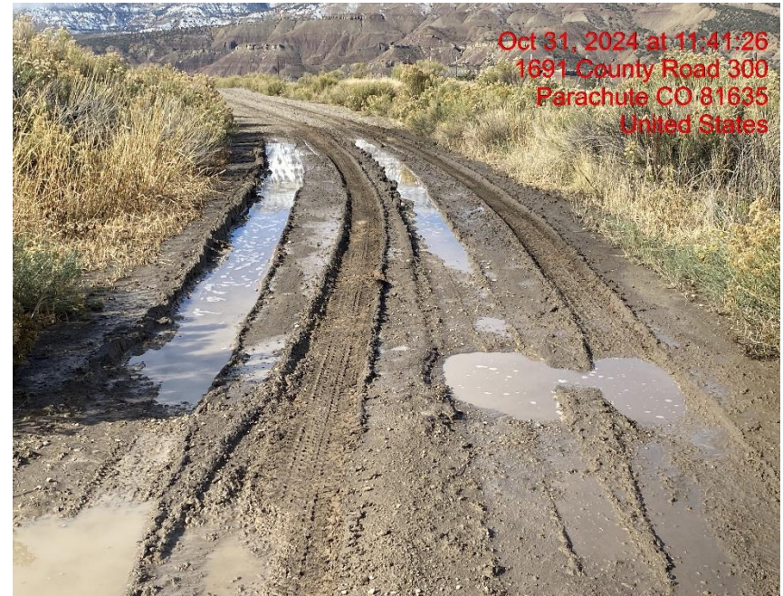
Lack of Stabilization on Access Road – Photo #04605
