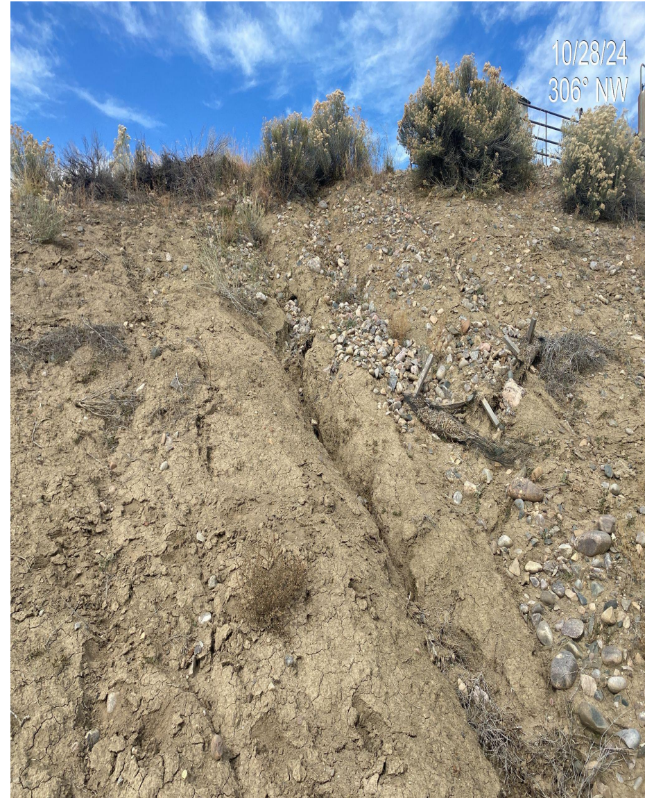
Photo 3. View of erosion and storm water BMPs that are no longer functioning in the eastern interim reclamation area.
