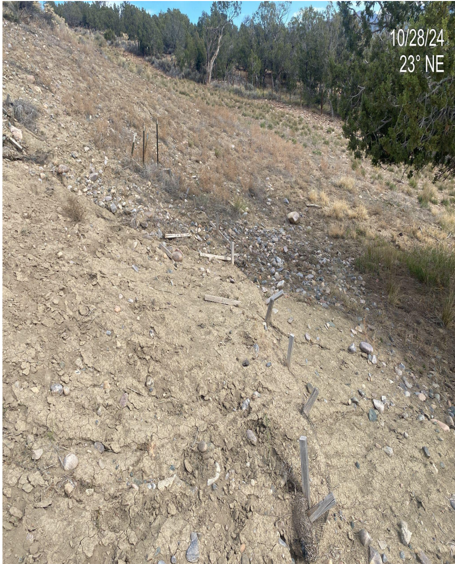
Photo 3. View of erosion and storm water BMPs that are no longer functioning in the eastern interim reclamation area.
