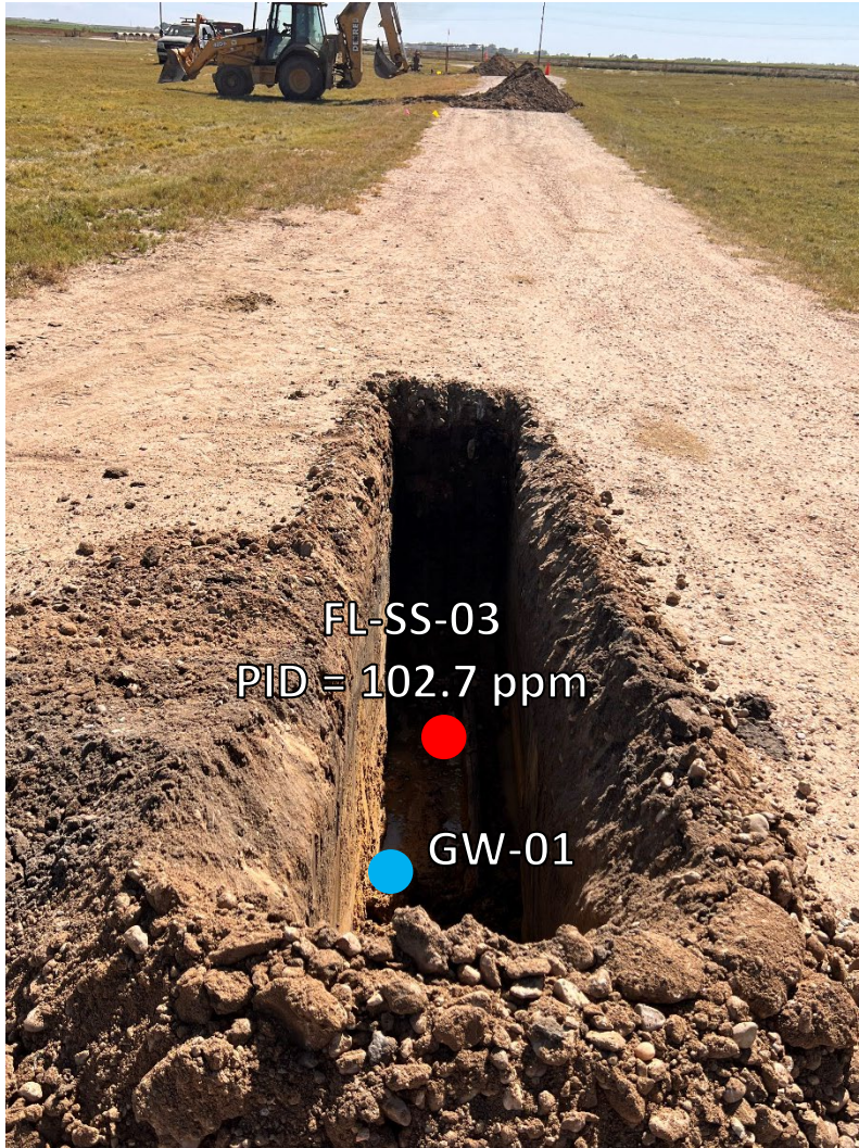
Looking south at bellhole/cut point for removal
