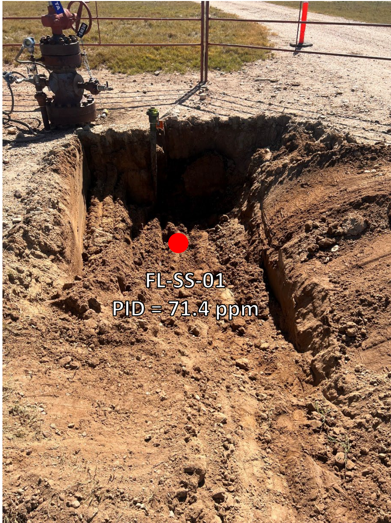
Looking southwest at flowline Pt A/terminus at wellhead
