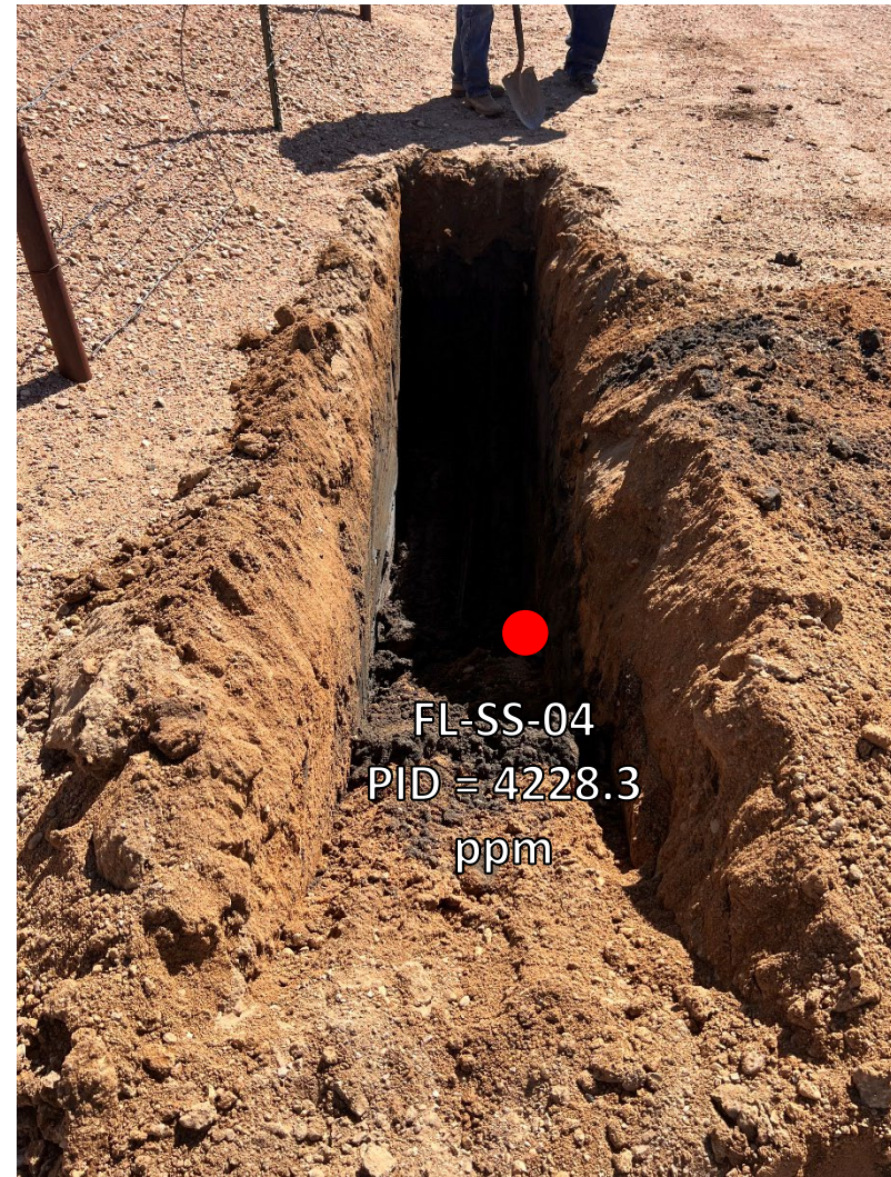
Looking south at bellhole/cut point for removal
