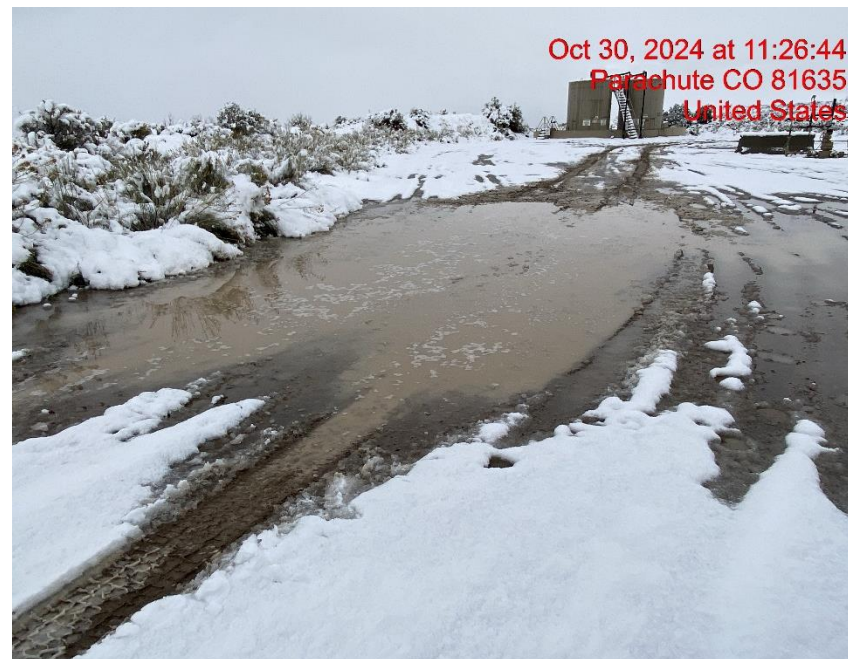
Lack of Stabilization/Standing Water – Photo #04583
