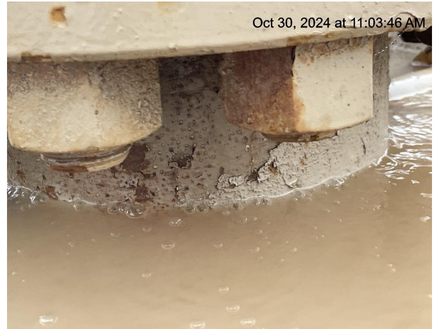
Photo # 8156 Possible wellhead leak/gas bubbling up through water around wellhead (FEDERAL RMV 63-19 well)
