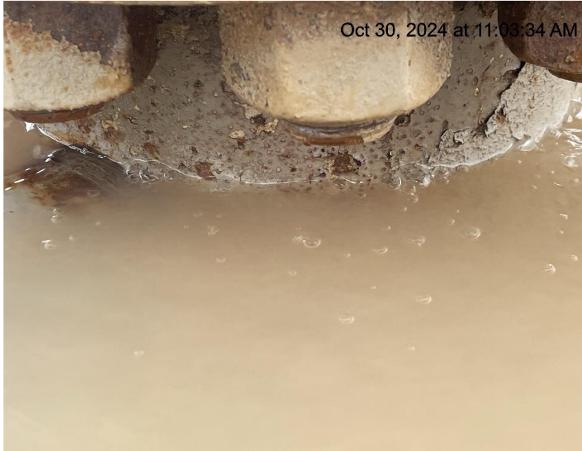
Photo # 8157 Possible wellhead leak/gas bubbling up through water around wellhead (FEDERAL RMV 63-19 well)
