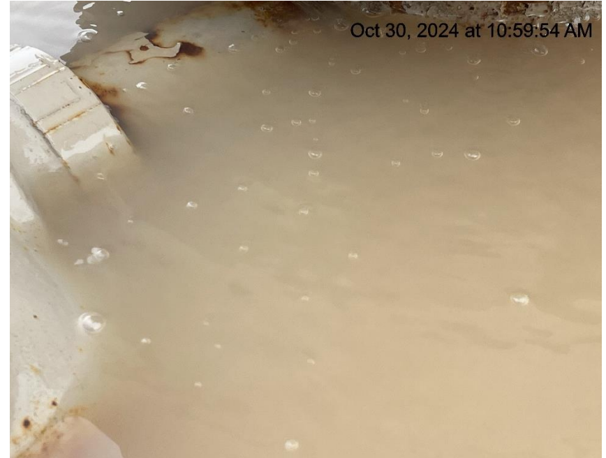
Photo # 8158 Possible wellhead leak/gas bubbling up through water around wellhead (FEDERAL RMV 63-19 well)
