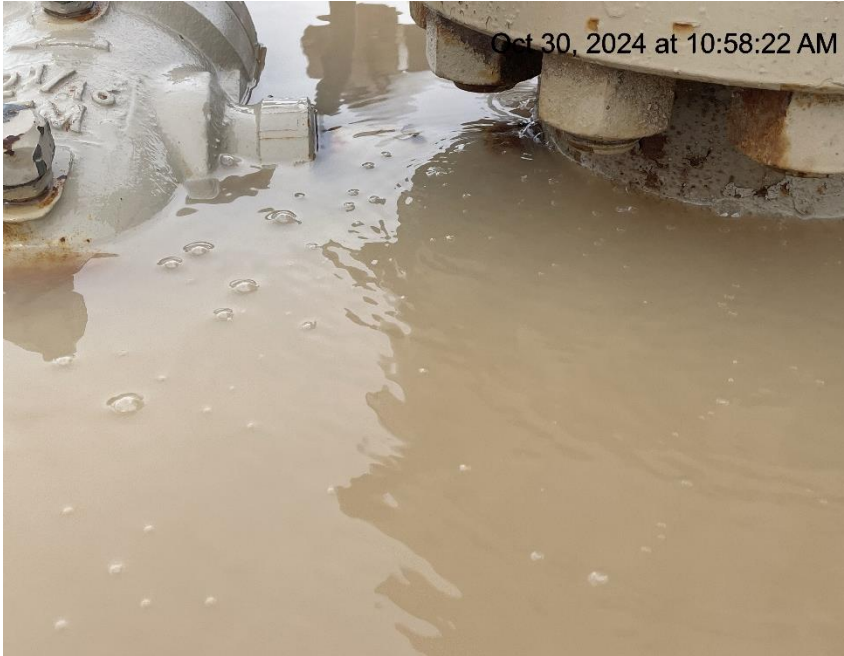
Photo # 8151 Possible wellhead leak/gas bubbling up through water around wellhead (FEDERAL RMV 63-19 well)
