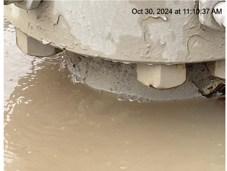
Photo # 8154 Possible wellhead leak/gas bubbling up through water around wellhead (FEDERAL RMV 63-19 well)
