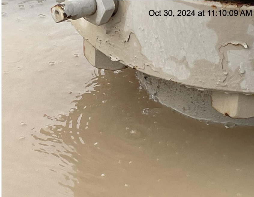
Photo # 8153 Possible wellhead leak/gas bubbling up through water around wellhead (FEDERAL RMV 63-19 well)
