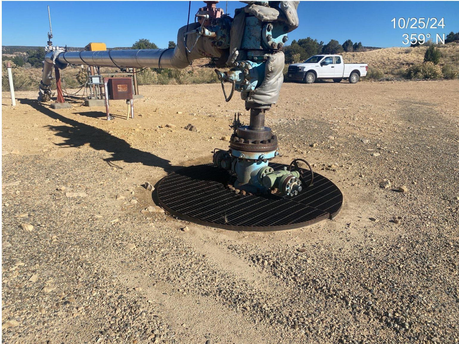
Photo 2. Gap in cellar grate was not observed during this inspection. Wildlife BMPs appear to be in working condition.
