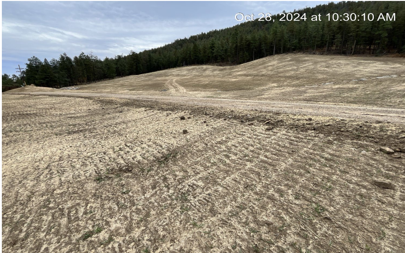
Photo 2. Facing southeast. The location has been recontoured and reclaimed. Soils have been tracked and lightly hydromulched.
