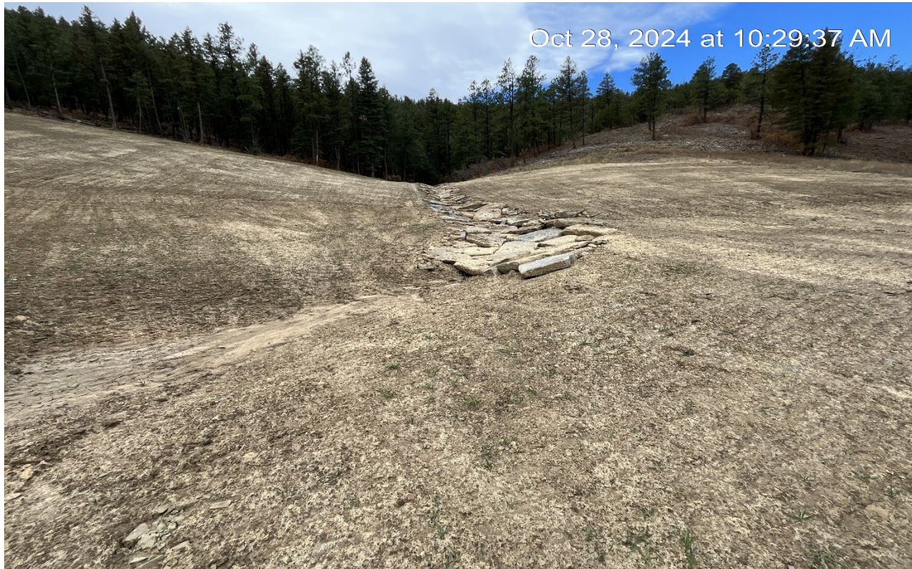
Photo 5. This drainage was stabilized with rock rip/rap for stormwater run-on..
