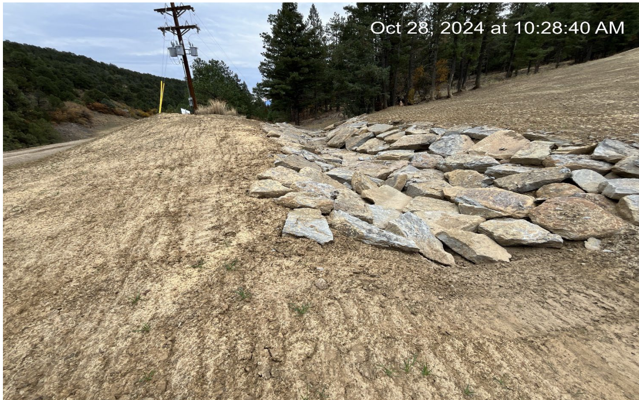
Photo 6. Facing toward the east side of the location. This rip/rap outlet appears to have too much rip/rap and may affect drainage as it appears to be slightly higher gradient.
