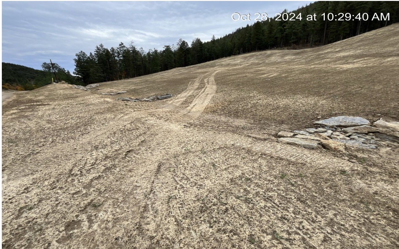
Photo 4. Facing east at the center of the location. A berm was installed with rock dams.
