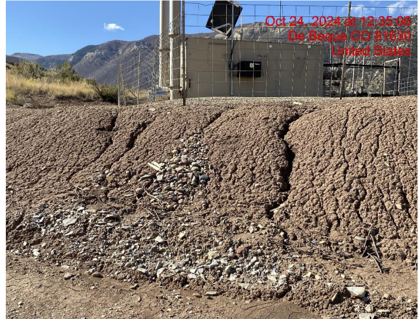
Rill Erosion/Sediment Transport Offsite – Photo #04498
