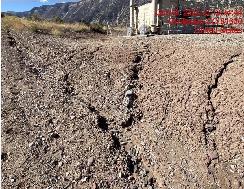
Rill Erosion/Sediment Transport Offsite – Photo #04497
