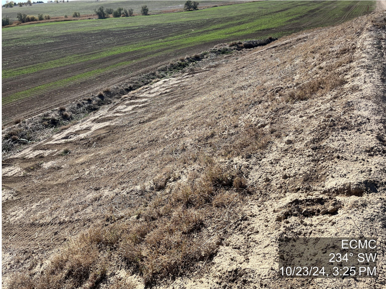
Photo 11. The photo was taken at the well location facing Southwest. The photo illustrates steep slopes along the pad edge have limited vegetation and stormwater controls.
