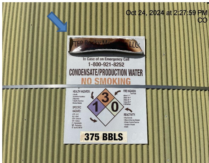
Photo # 7400 Some required info on tank label is weathered & illegible
