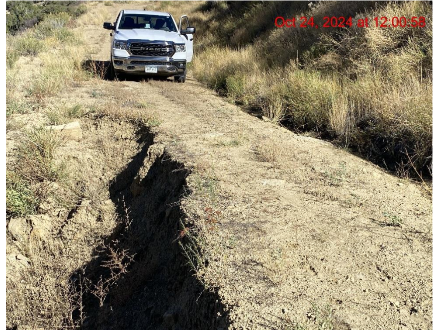
Location Inaccessible Due to Lease Road Slide – Photo #04468
