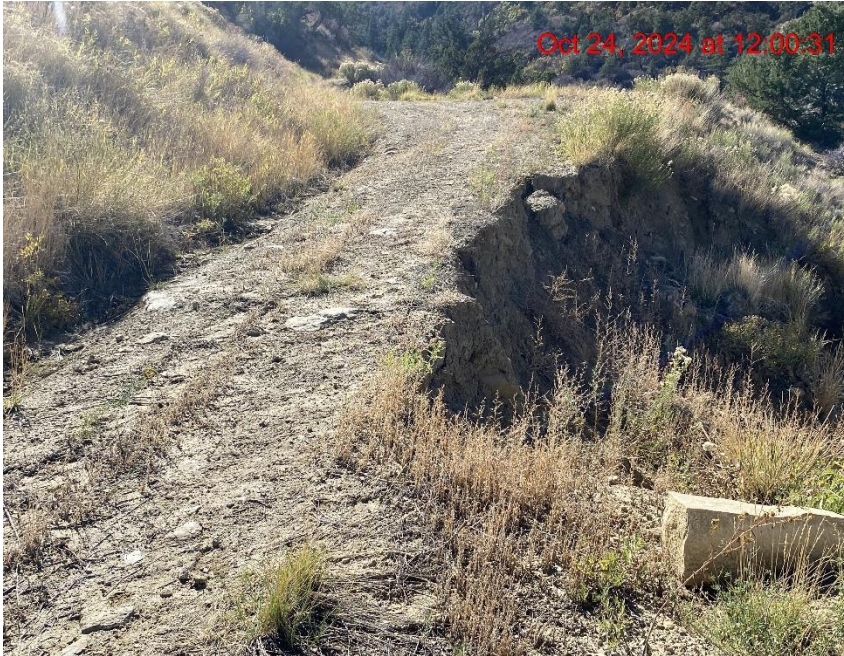
Location Inaccessible Due to Lease Road Slide – Photo #04467
