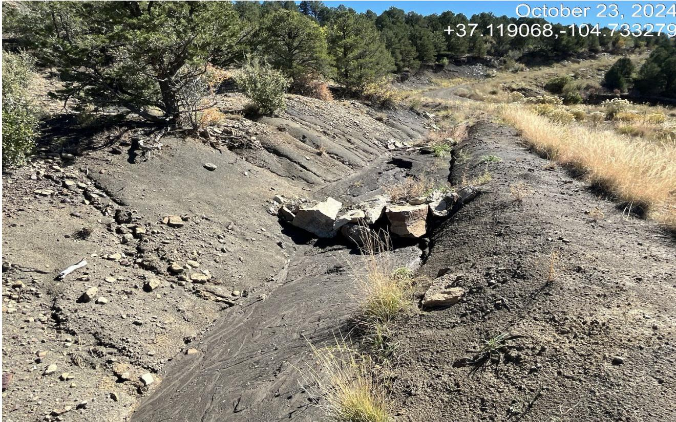
**Photo 6.** This run-on ditch from the road needs additional seeding and the check dams needs to be cleaned out.
