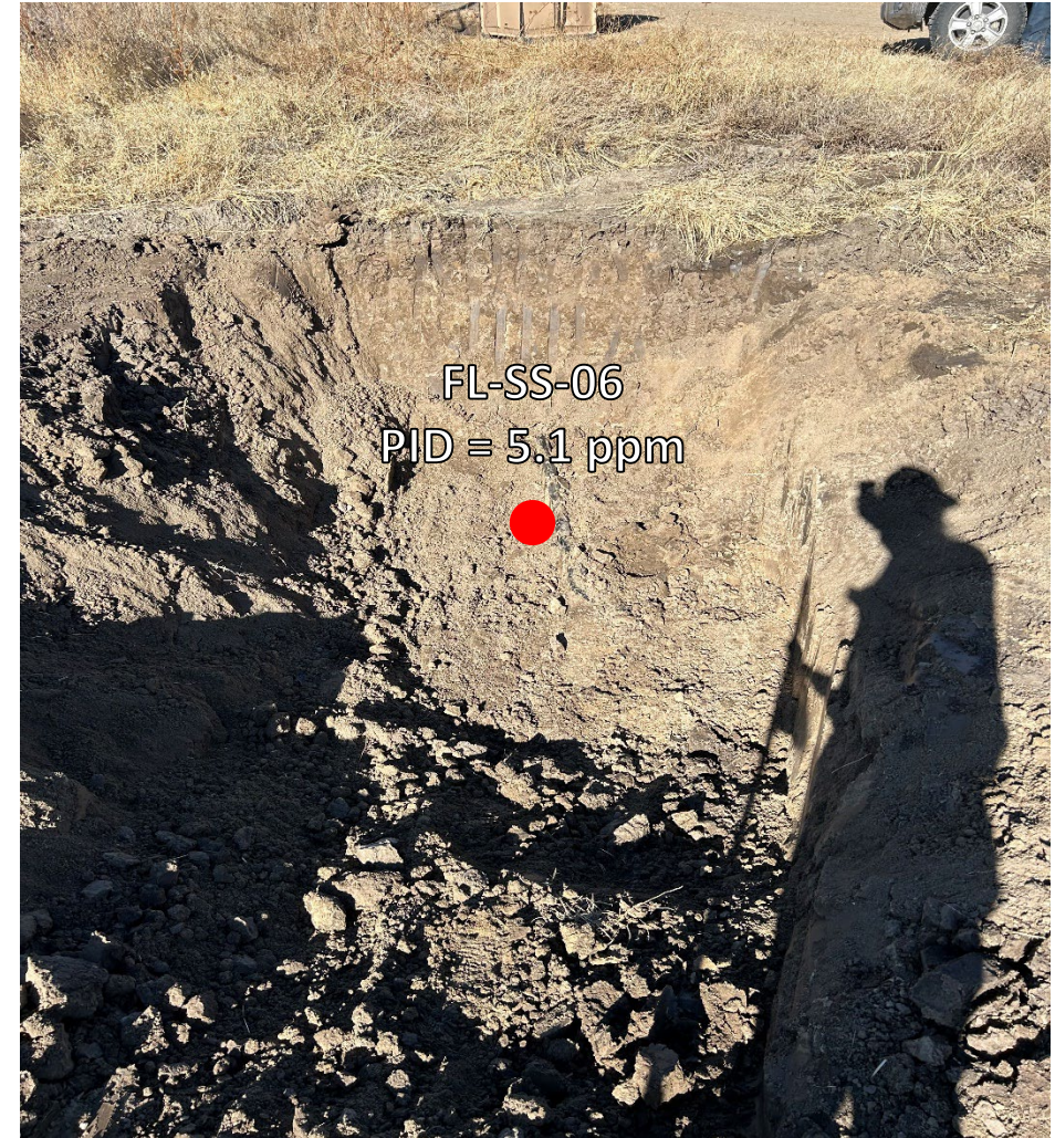
Looking north at flowline directional change
