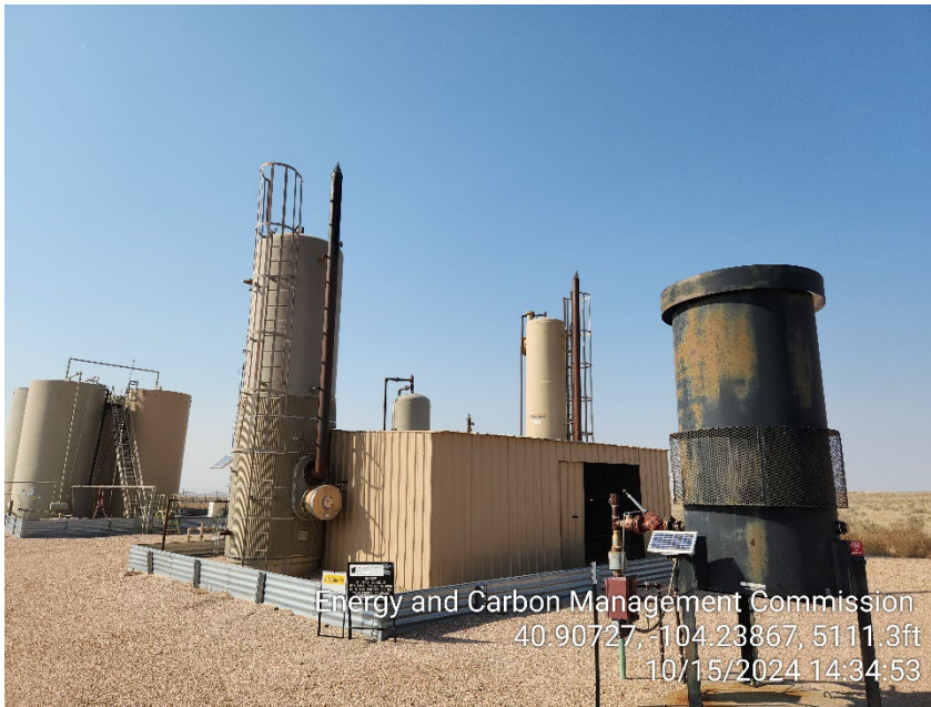
Photo 1 – Heater Treaters and ECD
