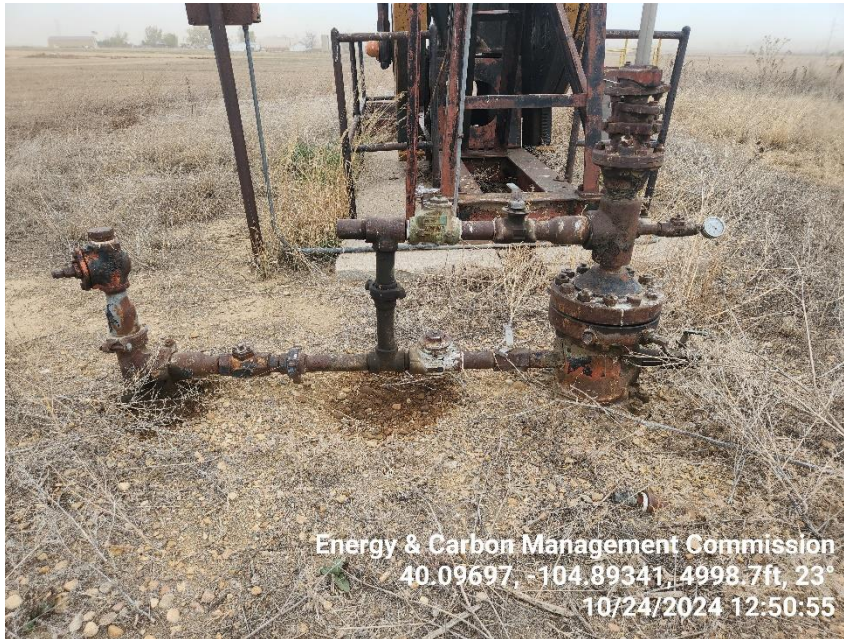
Photo 3 Stained Soil by the WH flow line.
