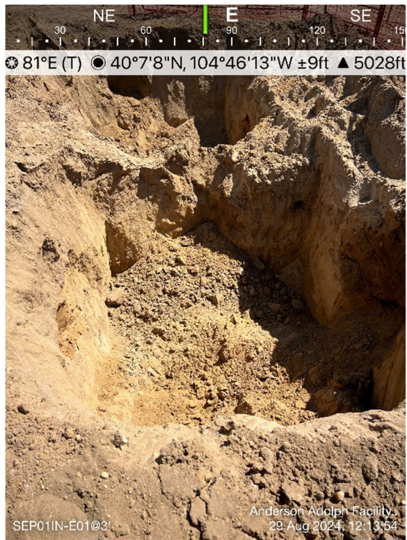
Separator Inlet Excavation
