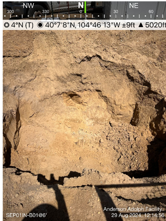
Separator Inlet Excavation
