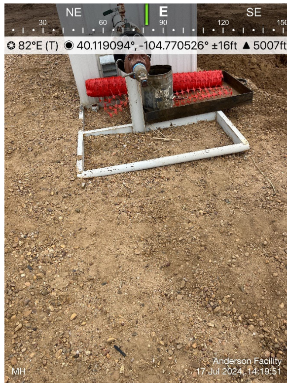
Meter House Location
