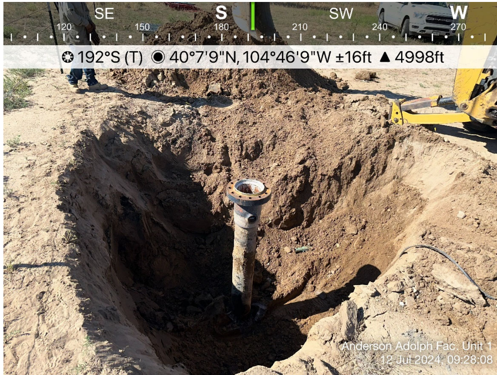
Wellhead Excavation
