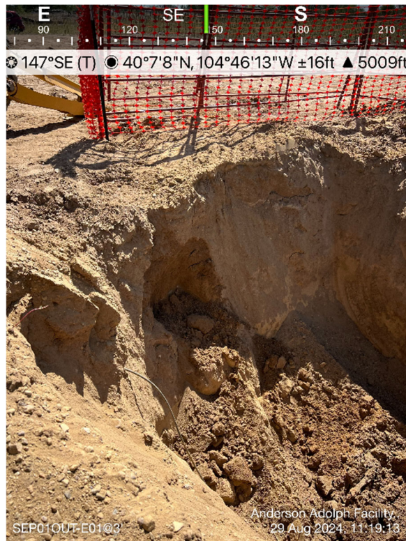
Separator Outlet Excavation
