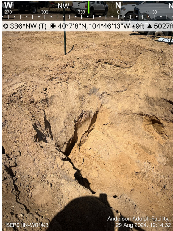
Separator Inlet Excavation
