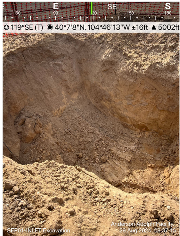
Separator Inlet Excavation
