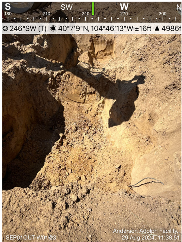
Separator Outlet Excavation
