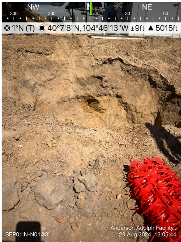
Separator Inlet Excavation
