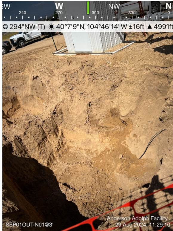
Separator Outlet Excavation
