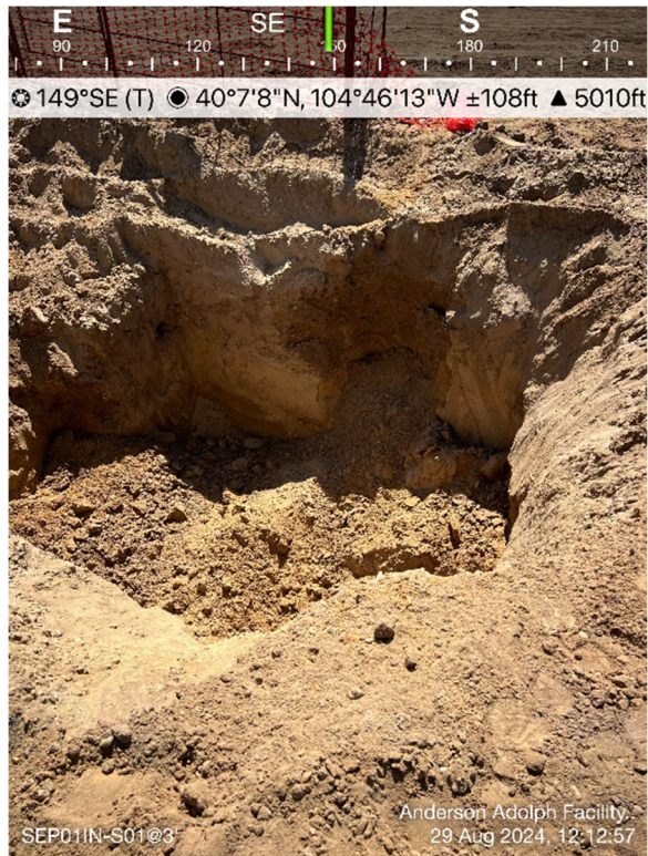
Separator Inlet Excavation
