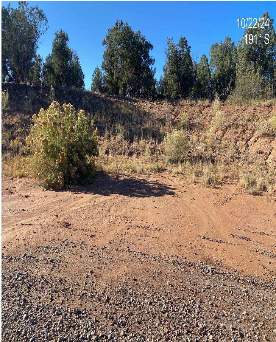
Photo 4. View of active erosion and sediment transport/deposition occurring in the SW corner of the location on the cut slope.
