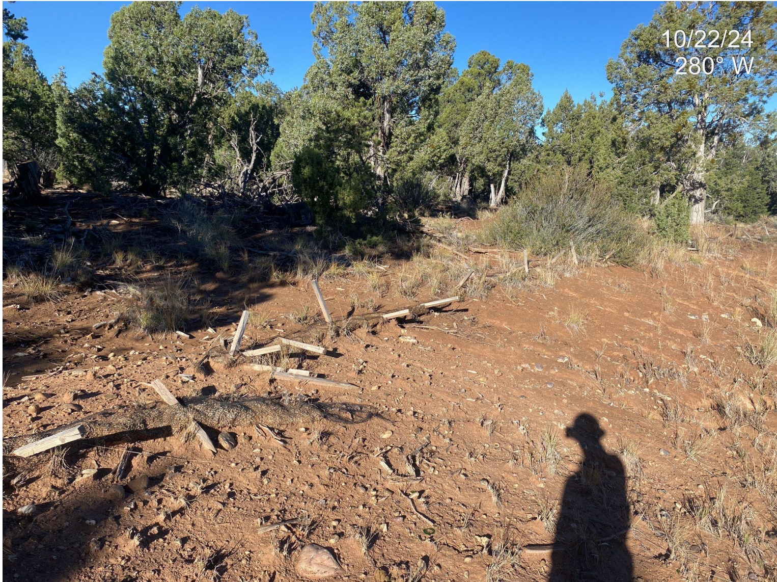
Photo 5. View of perimeter wattles that are damaged and no longer functioning, maintenance is needed in this area.
