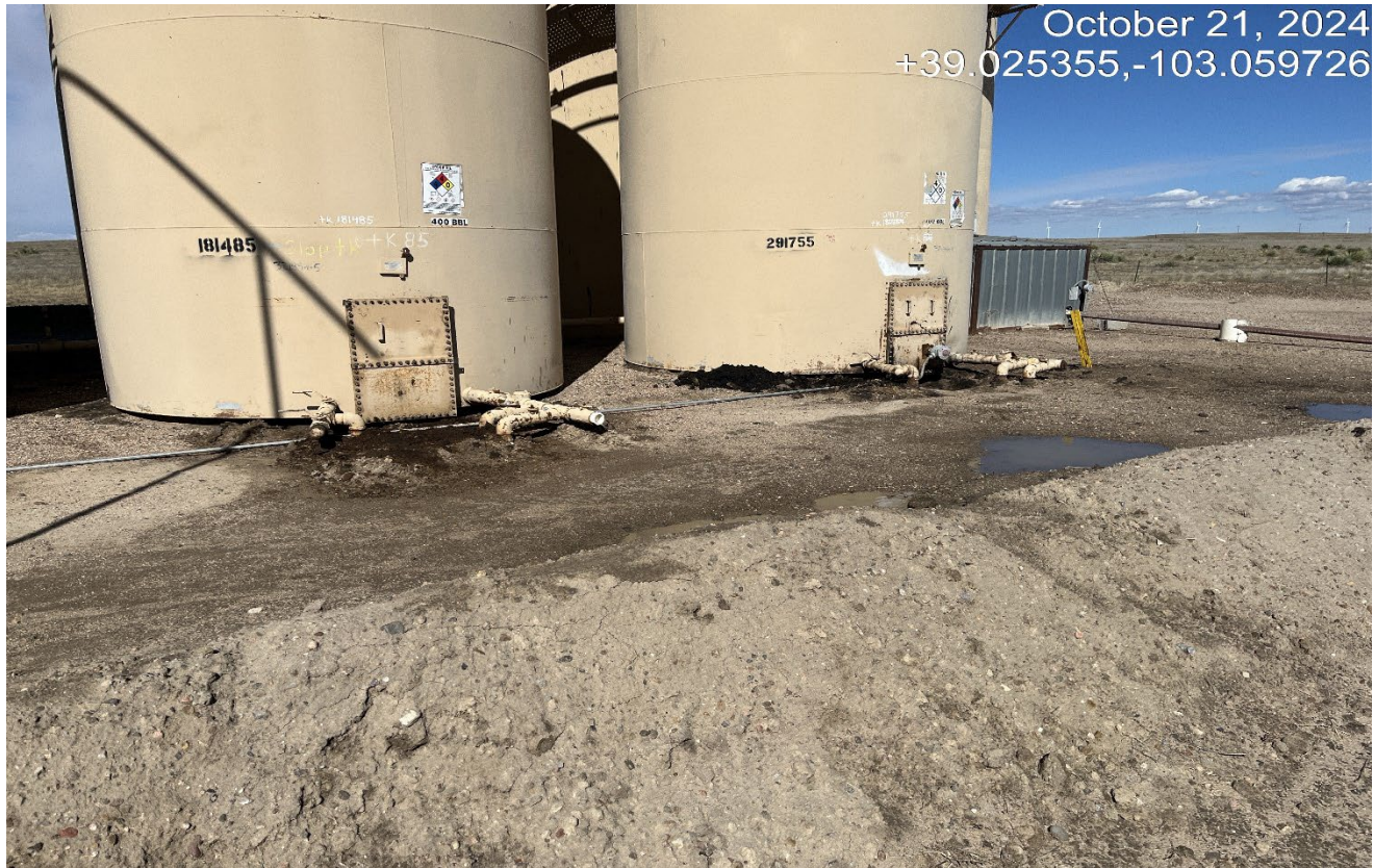
Photo 3. There are oil stained soils at the base of these tanks that need to be cleaned up.
