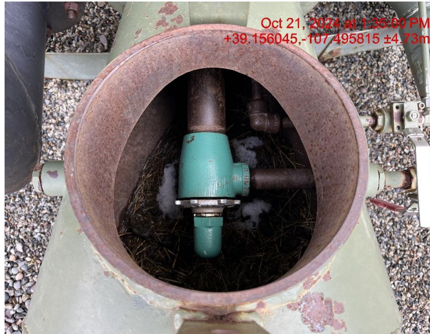
Photo # 7723 Tank heater open to wildlife hazard/ available for entry by wildlife
