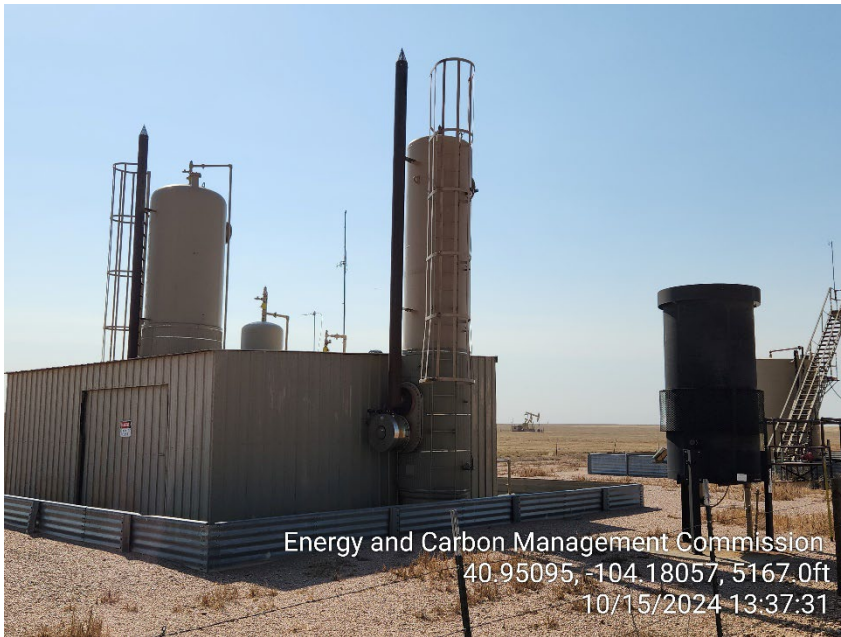
Photo 1 – Heater Treaters and ECD
