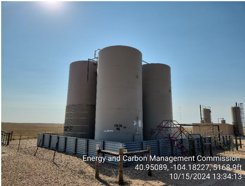
Photo 1 – Tank Battery
