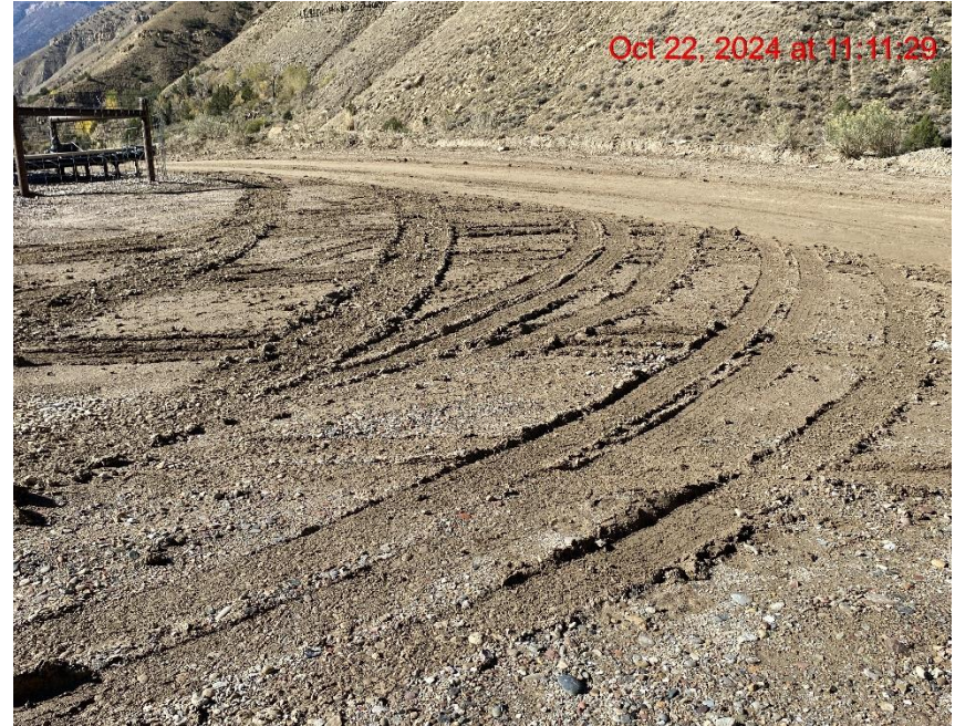
Insufficient Tracking BMPs – Photo #04340
