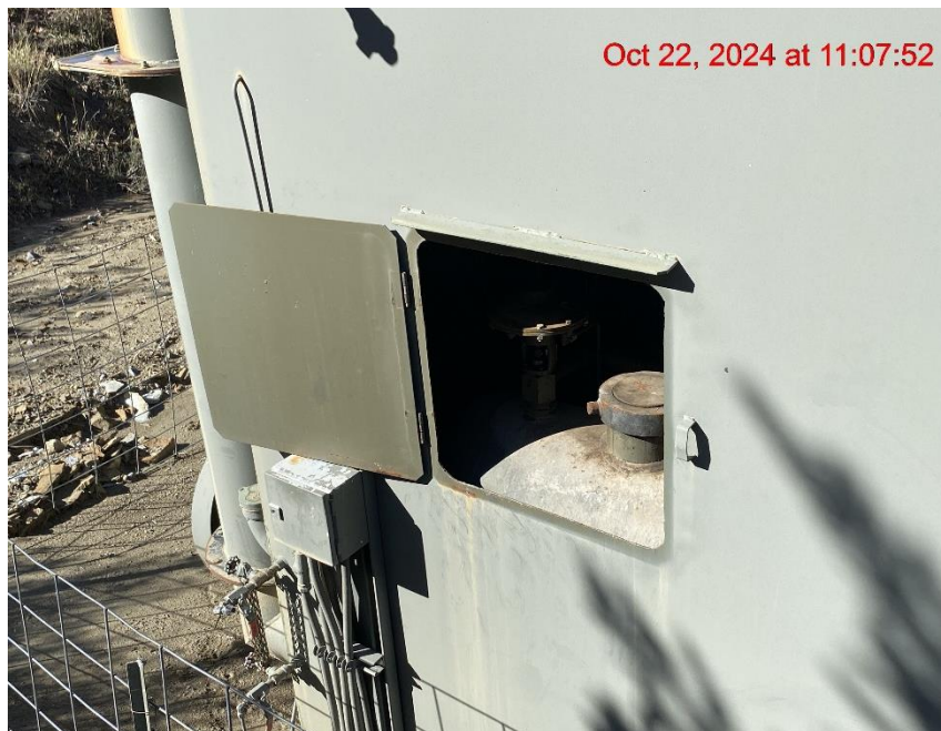
Unsecured Separator – Photo #04330
