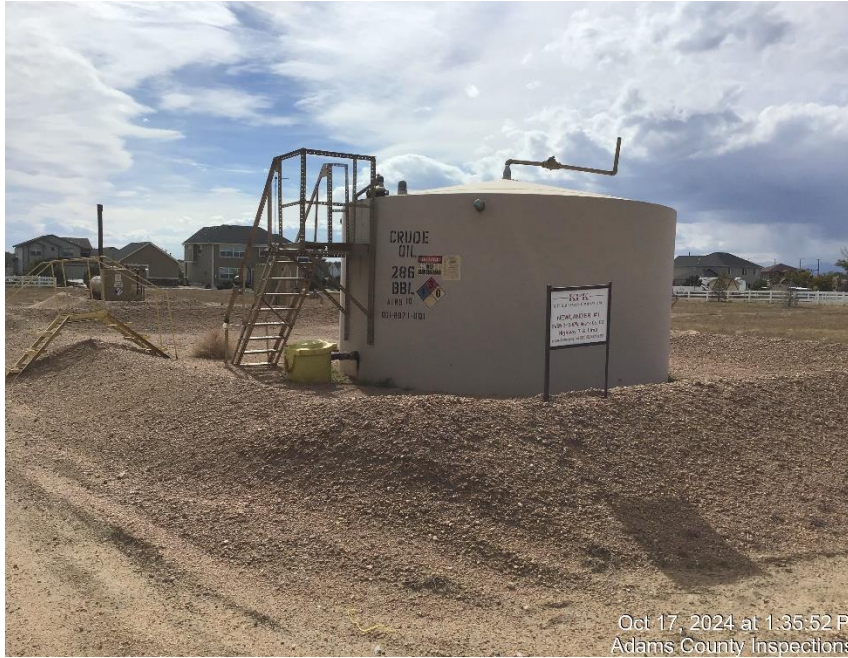
Photo #1 Crude tank.
