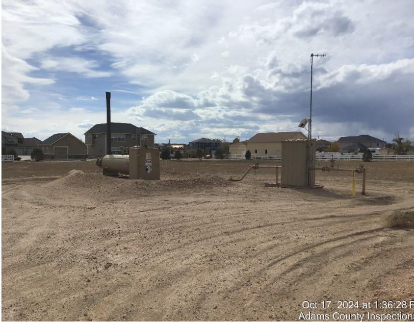
Photo #3 Separator and meter run.
