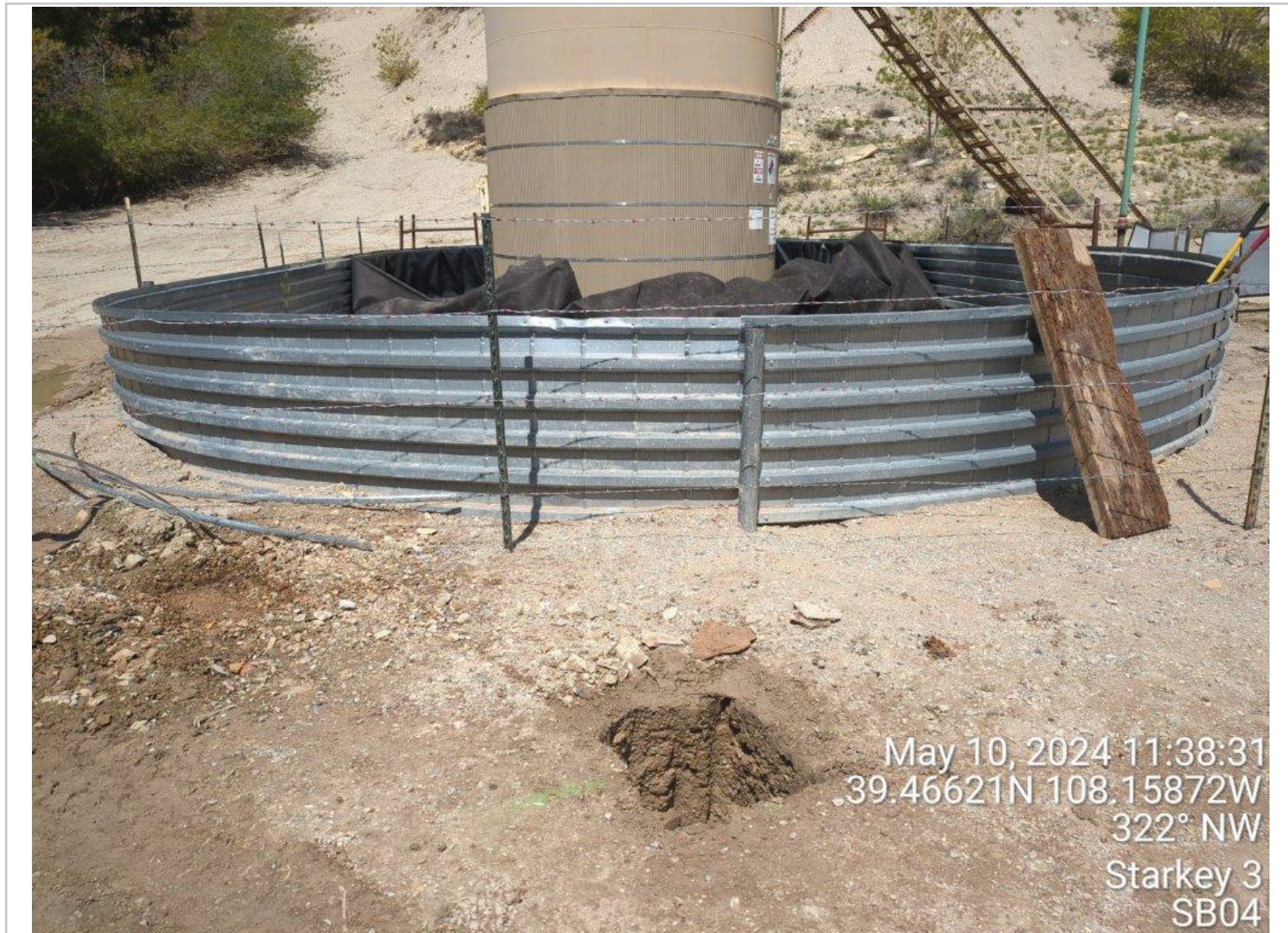
SB04: View Northwest
