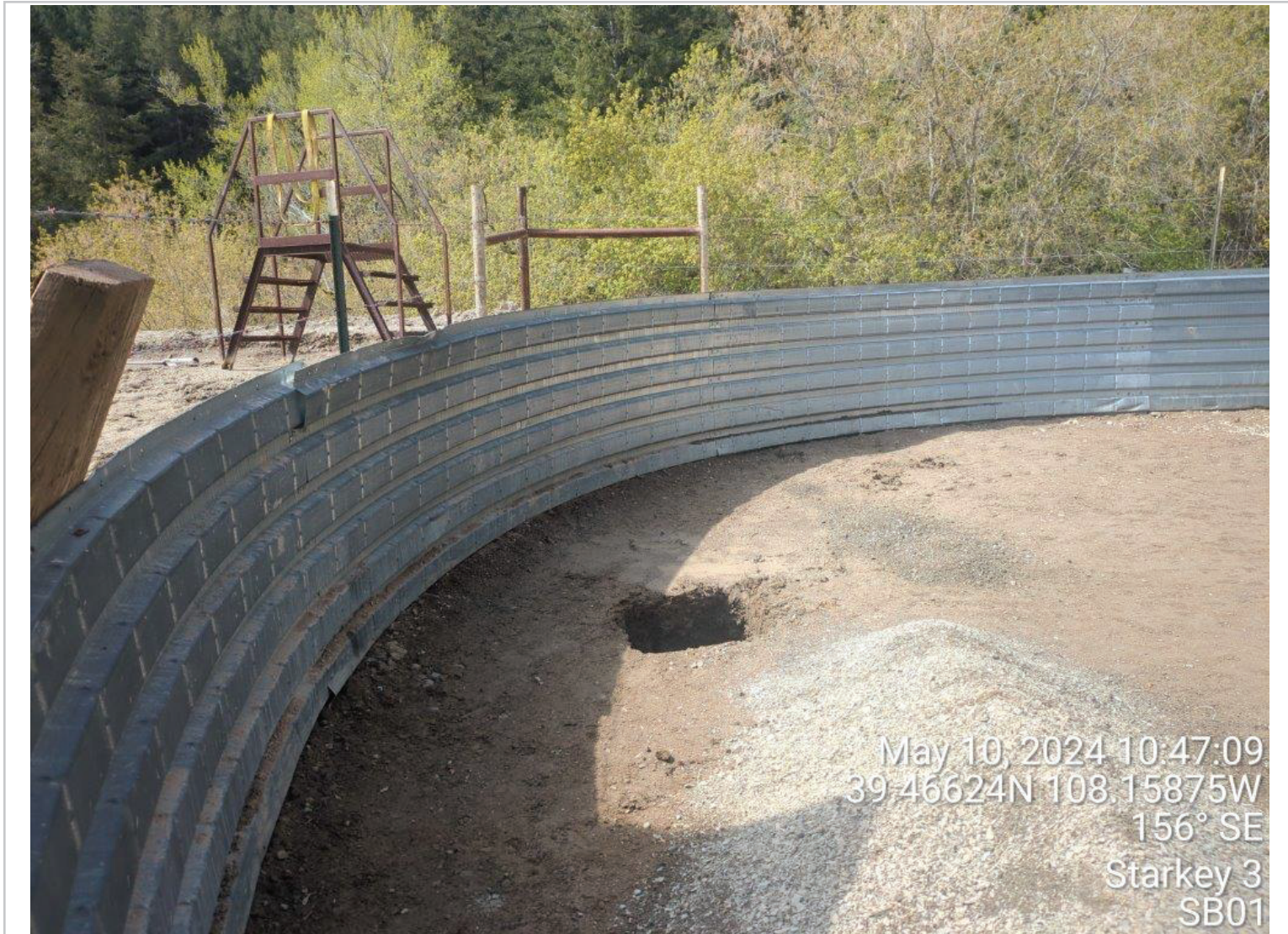
SB01: View Southeast
