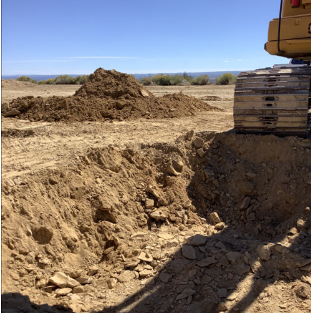
Photo 7: Meter house excavation and stockpile
