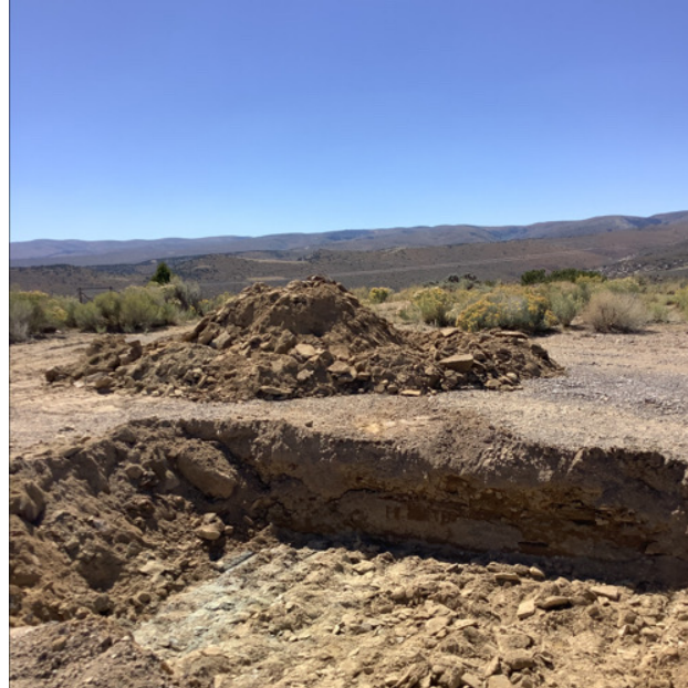
Photo 5: Separator excavation and stockpile
