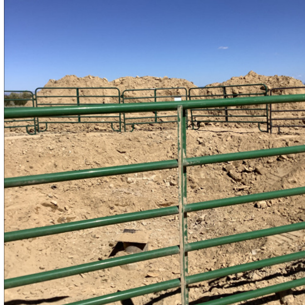
Photo 8: Wellhead excavation and stockpile
