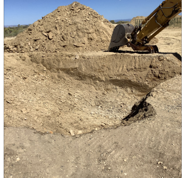
Photo 6: T03 excavation and stockpile
