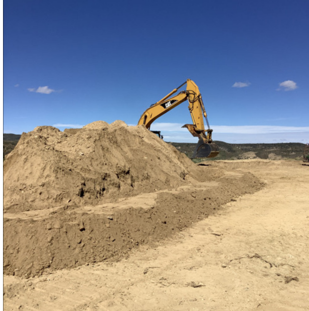
Photo 5: Stockpile associated with Pit excavation facing west
