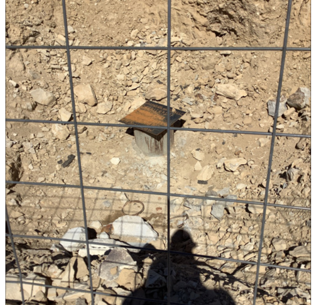
Photo 6: Capped wellhead at 5 feet bgs
