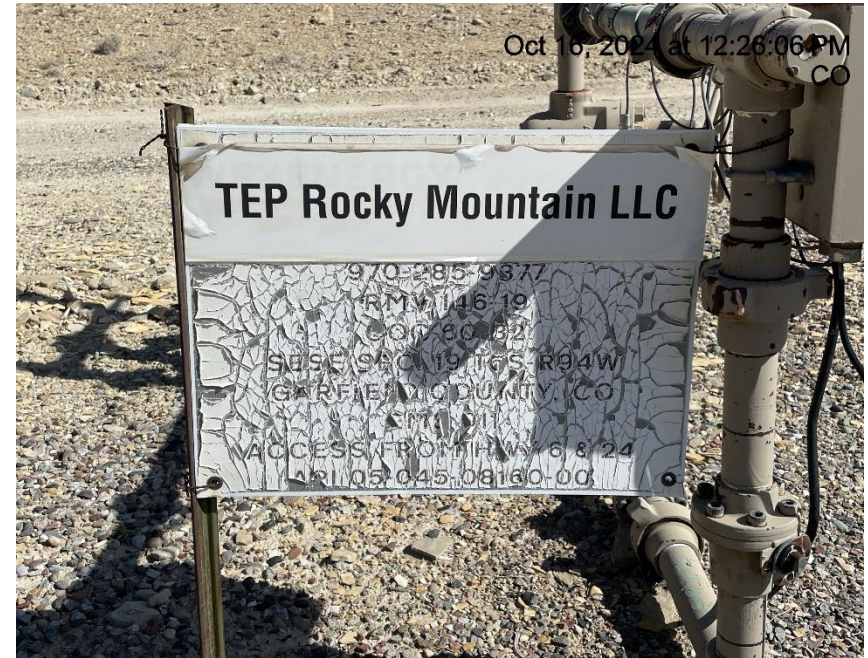
Photo # 6004 RMV 146-19 wellhead sign cracking & peeling/some required info starting to become illegible
