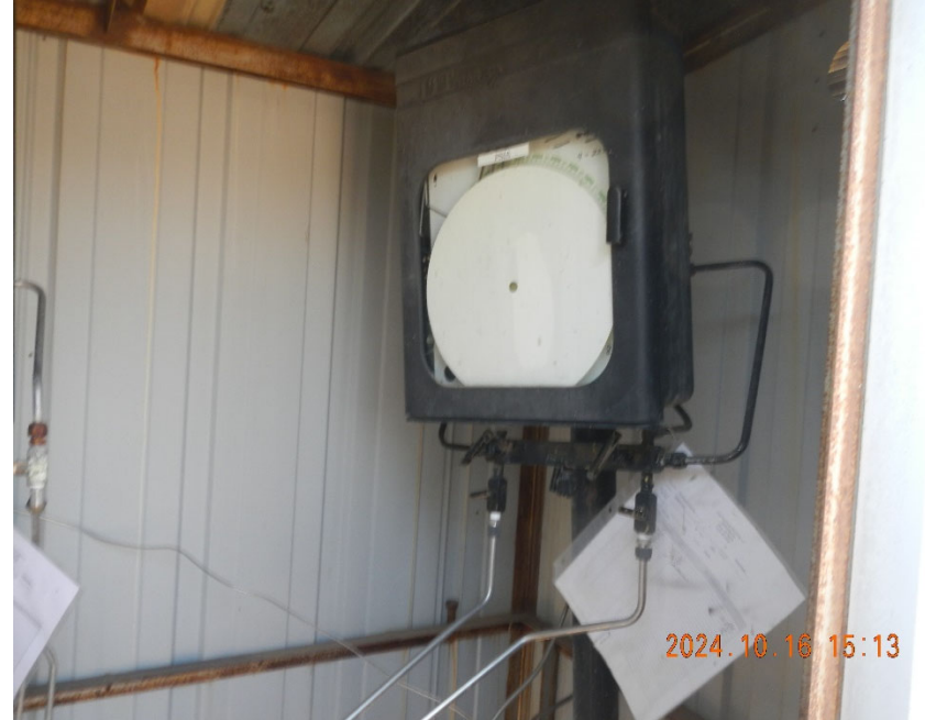
6. Gas meter inside shared meter shed.
