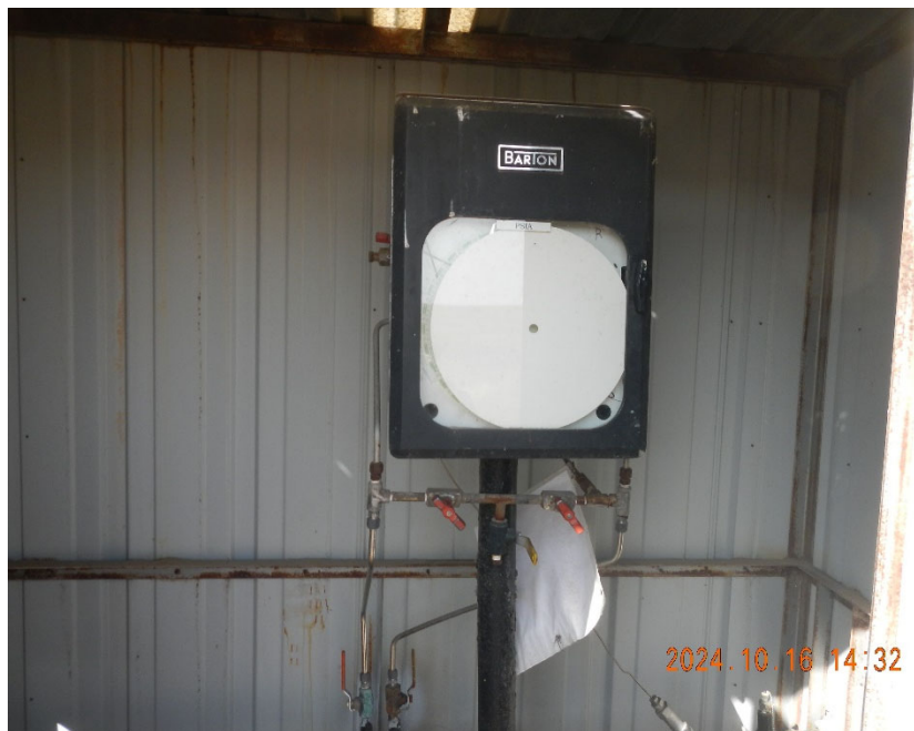
5. Shared Gas meter inside meter shed.
