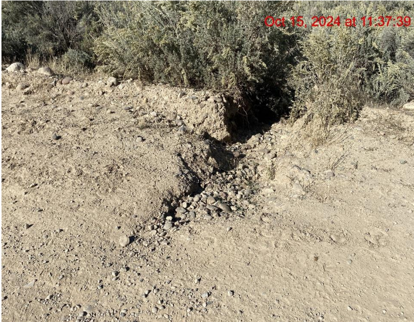
Insufficient Erosion Control/Sediment Transport from Lease Road – Photo #04237
