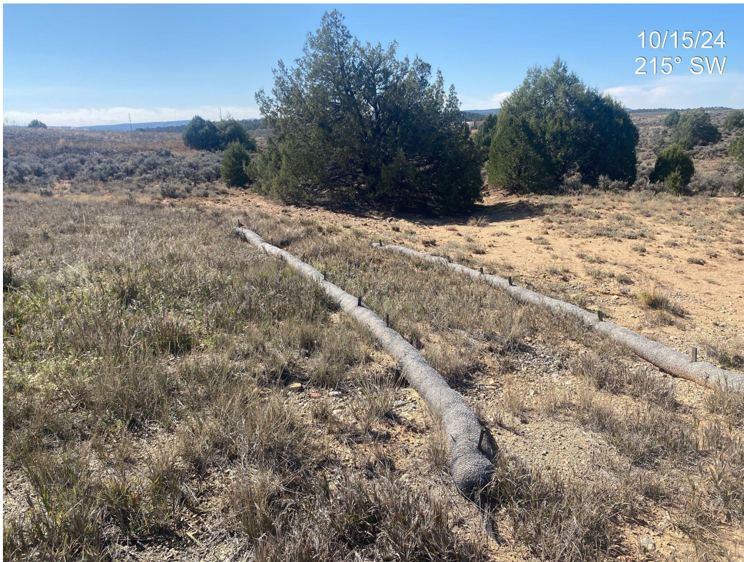
Photo 3. View of stormwater BMPs installed in the western portion of the disturbance. Erosion appears to be controlled at this time.
