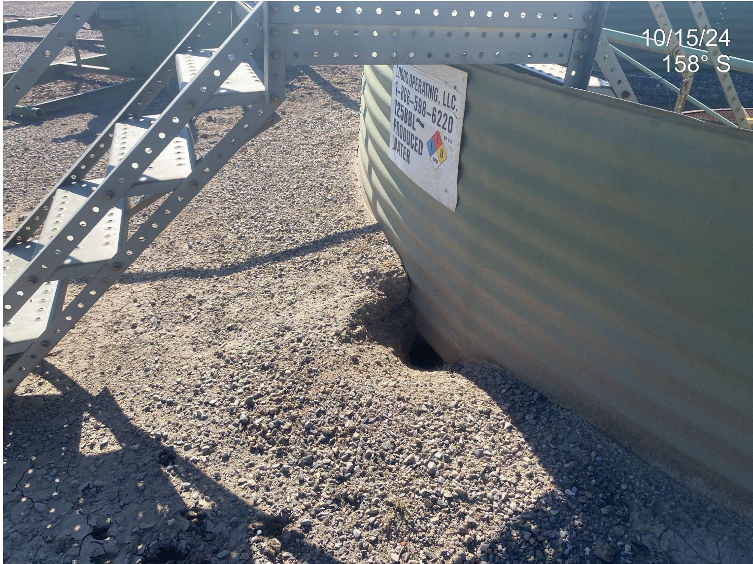
Photo 2. Animal burrow impacting produced water tank secondary containment.
