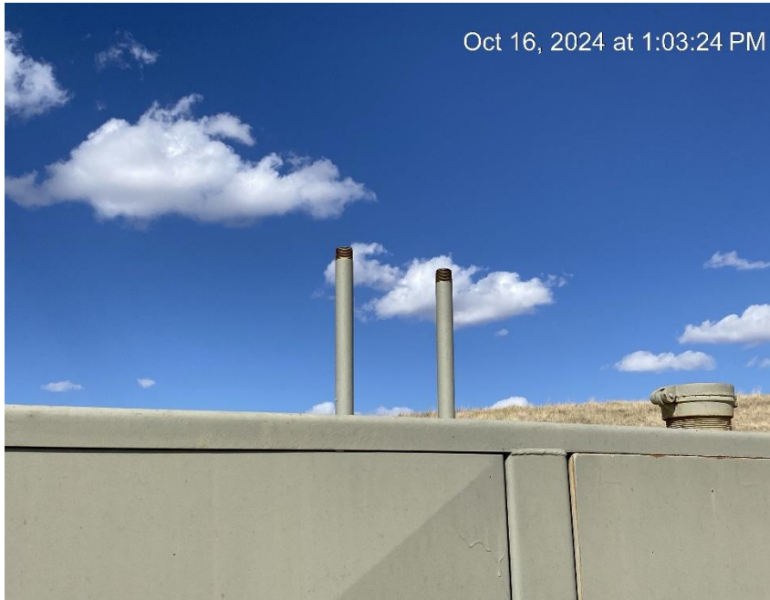
Unprotected vent risers
